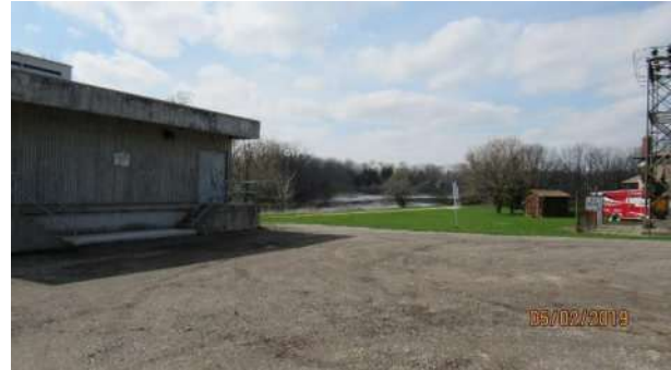
Plate 2: West view of pumping station and waterfront path; area beyond previous assessment requires Stage 2 survey
