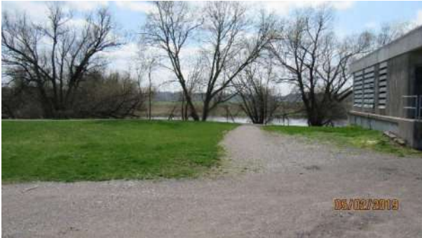
Plate 1: Southwest view of pumping station and waterfront path; area beyond previous assessment requires Stage 2 survey
