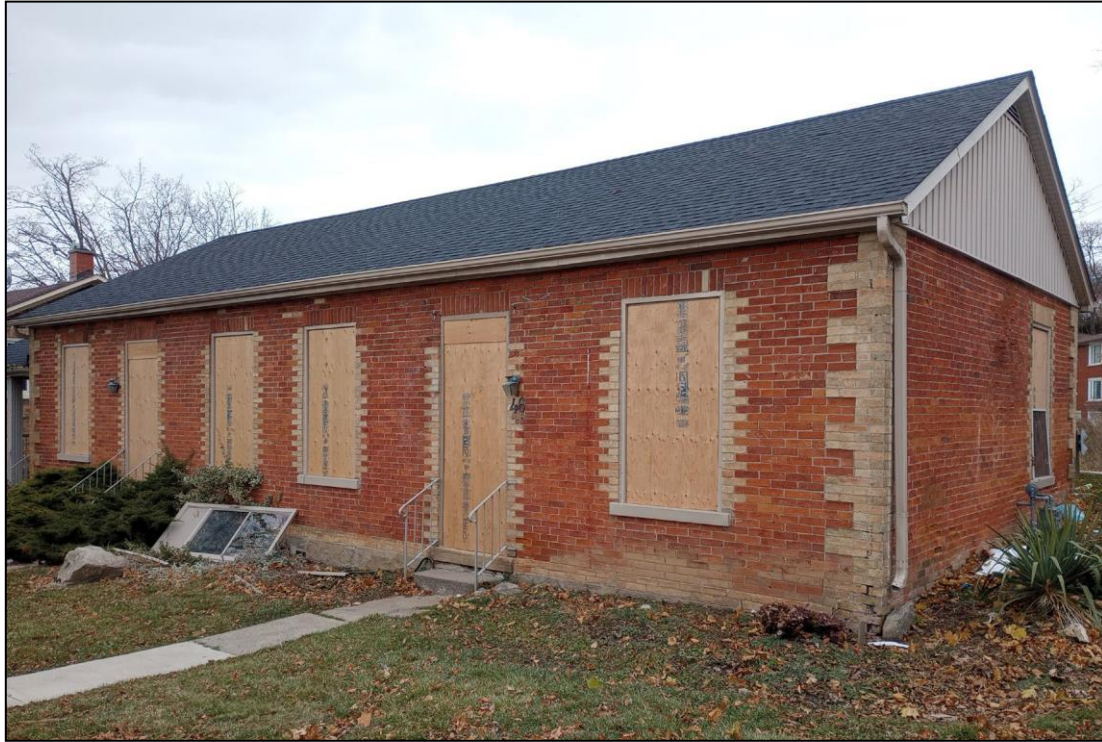
Figure 2: A view of the subject property from the southwest corner, at the intersection of Park Hill Road East and Cambridge Street, showing exterior details including dichromatic brickwork and raised quoins (City of Cambridge).
