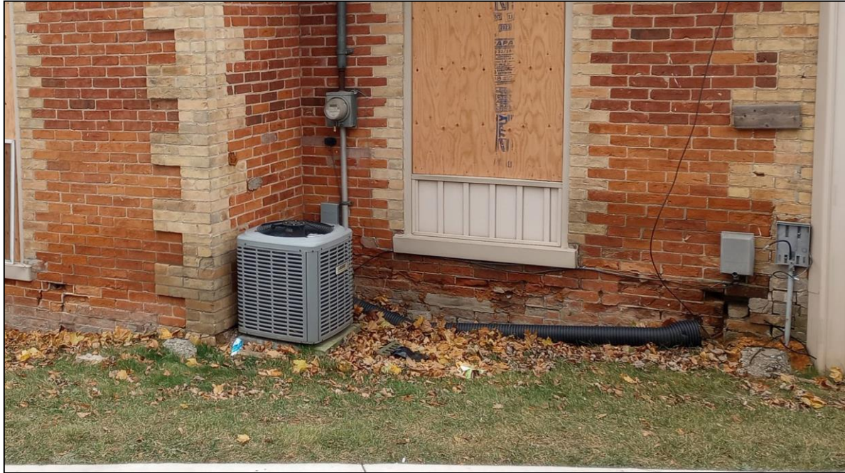
Figure 4: Showing brick spalling and degradation near foundation level (City of Cambridge).
