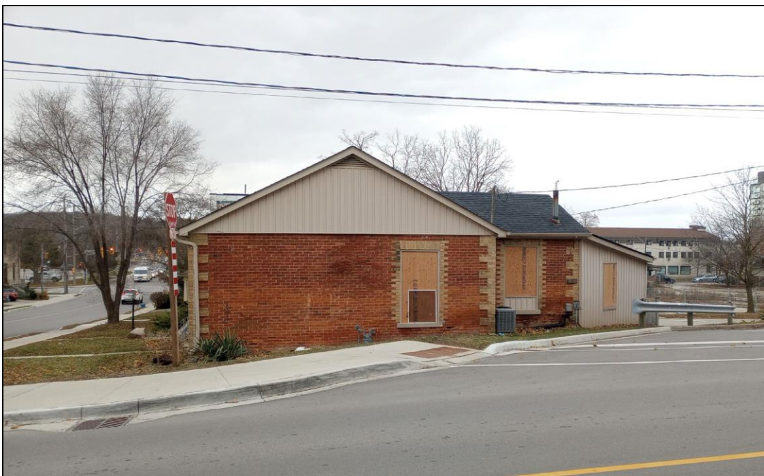
Figure 3: Looking west, showing the rear brick extension and small frame addition. The gable ends appear to be clad in modern vinyl siding (City of Cambridge).
