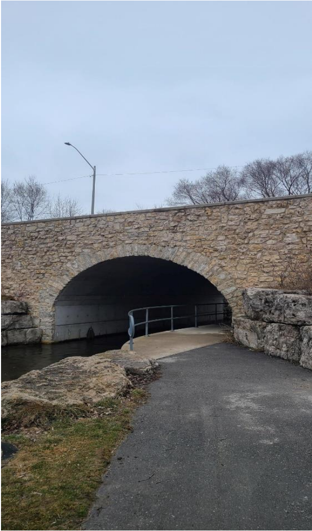
Figure 2: Stone arch over the Mill Creek, 2023
