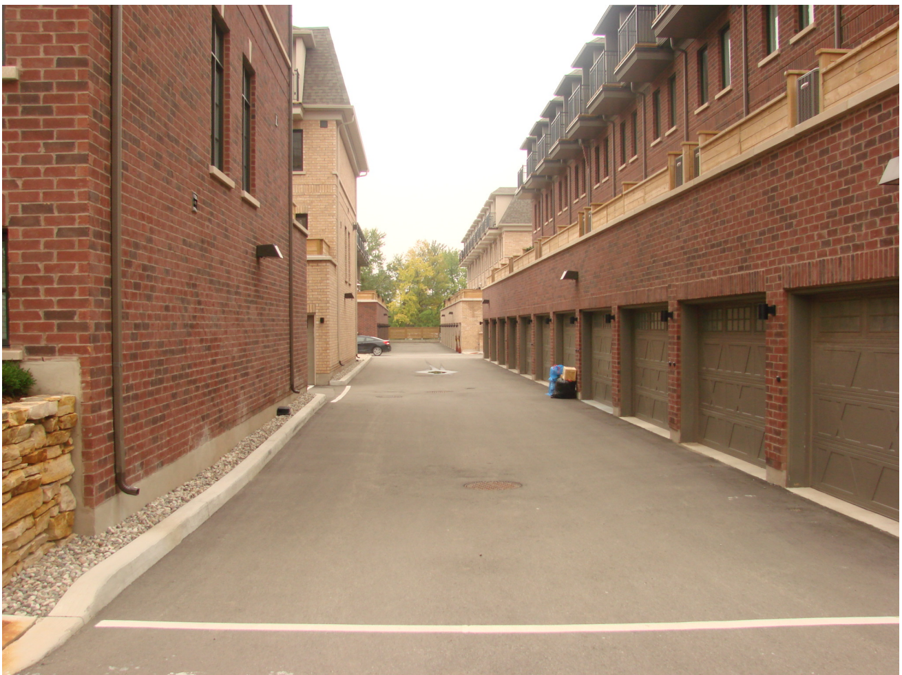
Figure 3: Sample of 8m Central Driveway
