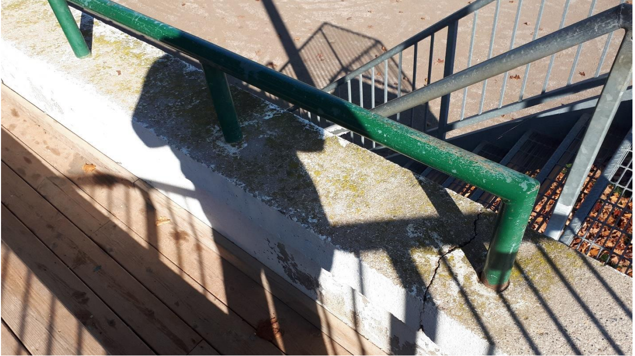
Figure 5: Image showing the condition of concrete walls and steel barriers proposed for repair and replacement (City of Cambridge).
