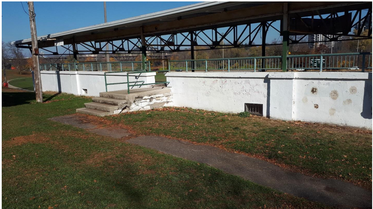
Figure 2: Rear of the grandstand structure showing deteriorated concrete steps (City of Cambridge).
