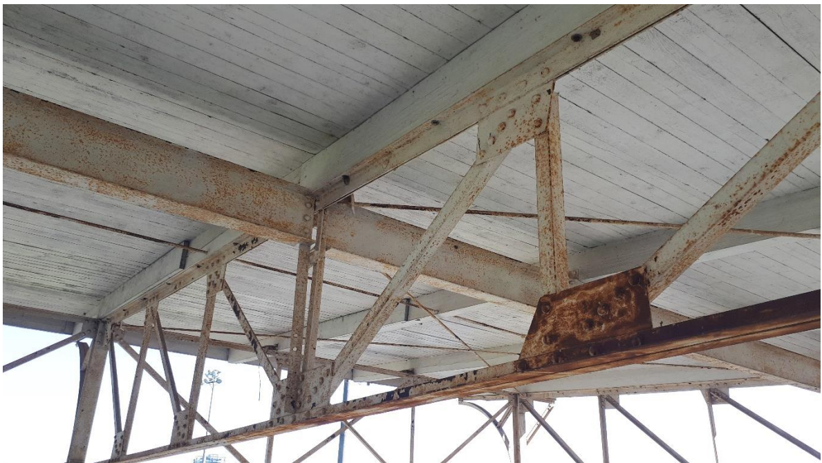
Figure 4: Looking up inside the grandstand structure to riveted steel roof trusses, beams, and wooden roof underlay (City of Cambridge).
