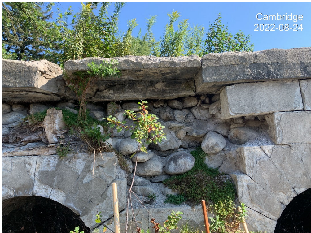
Photo 4 – Significant Exposure of Core of the North Stop Log Structure
