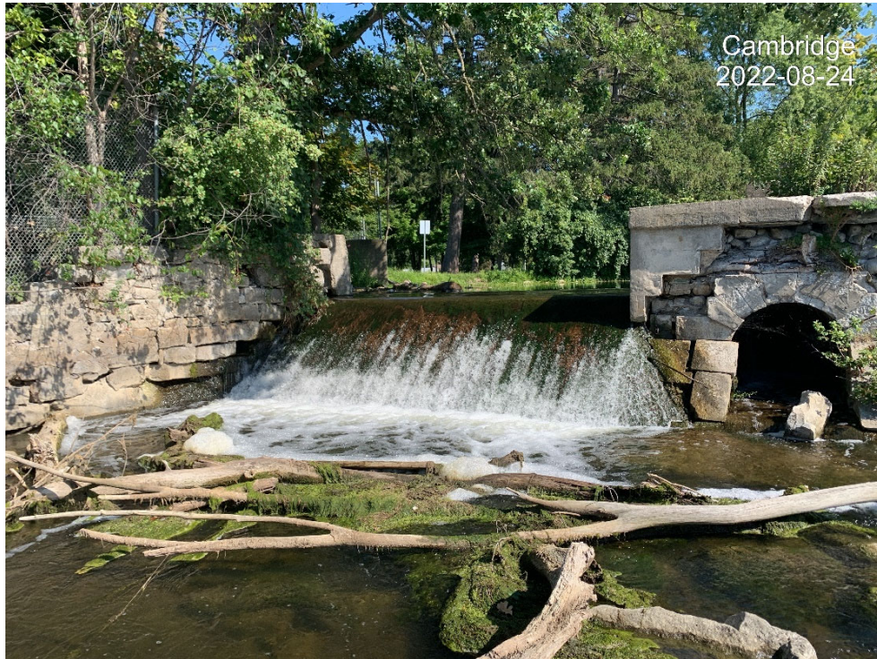
Photo 9 – North Retaining Wall / Loss of Concrete Cover and Mortar - No noticeable change since 2018
