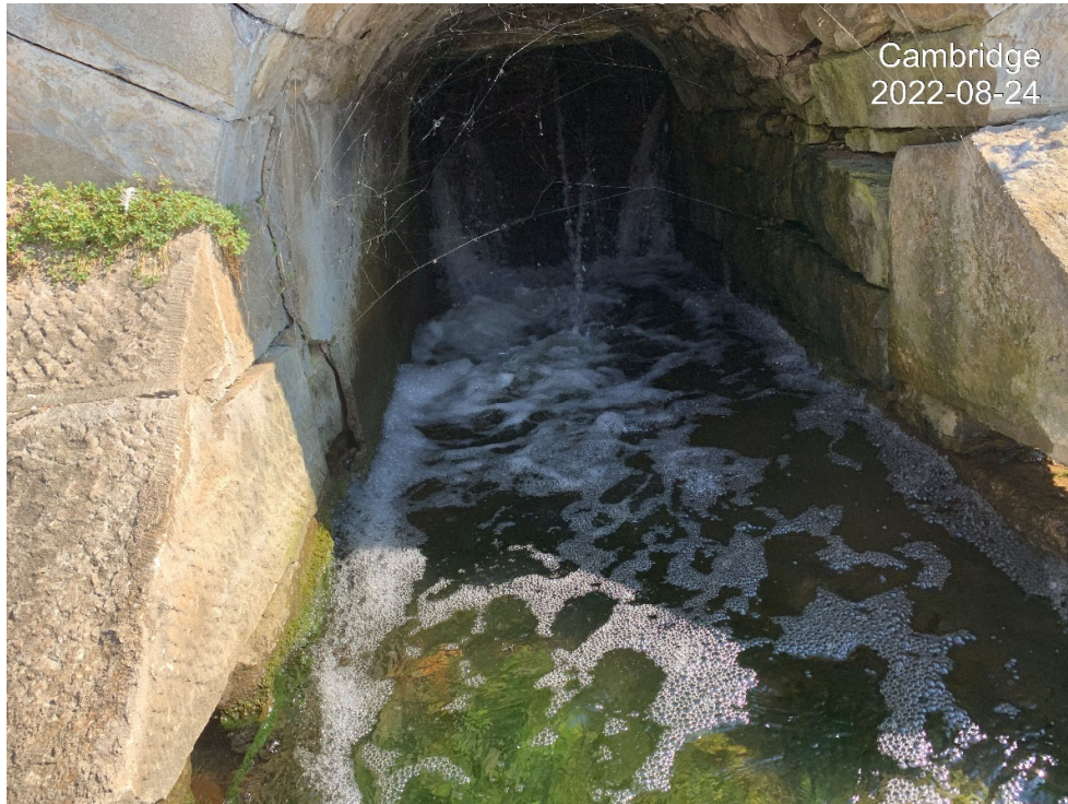
Photo 5 – Leaking Timber Stop Logs on Left Raceway of North Stop Log (Note the Exposed Masonry Blocks)
