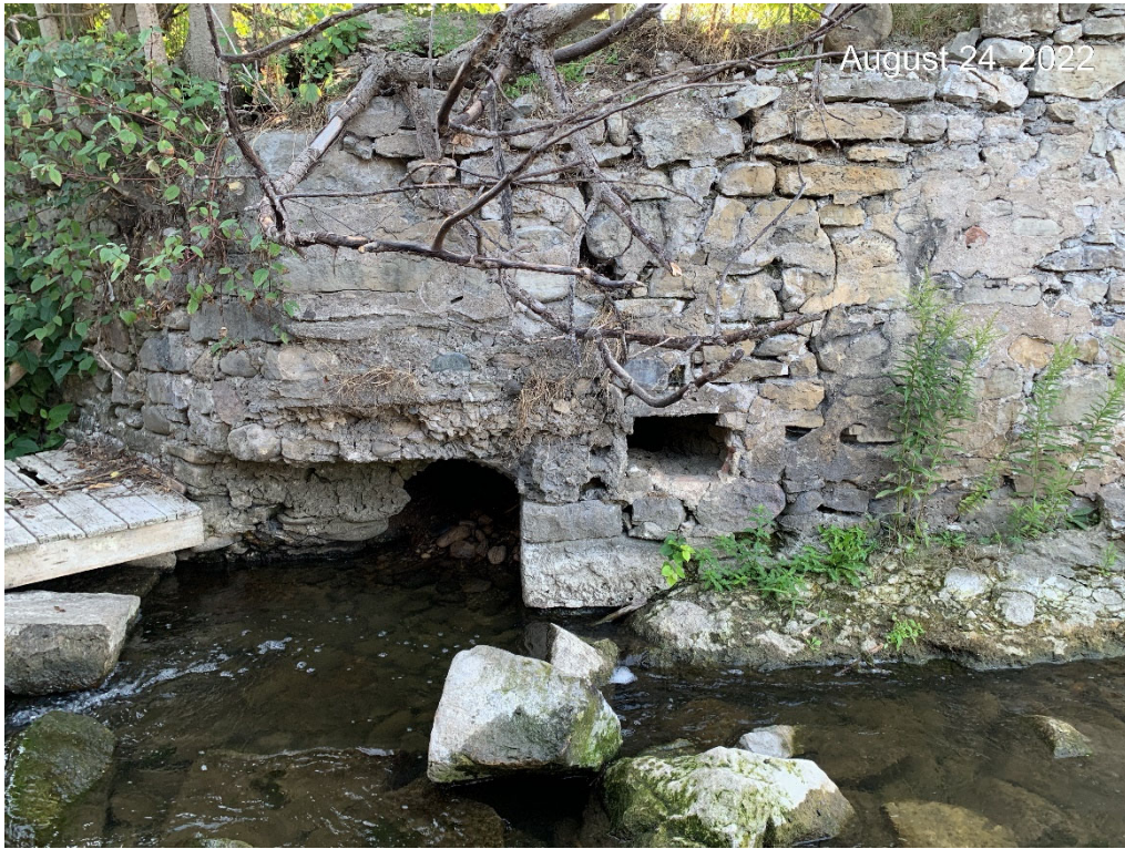
Photo 17 - Severe erosion and loss of material behind retaining wall
