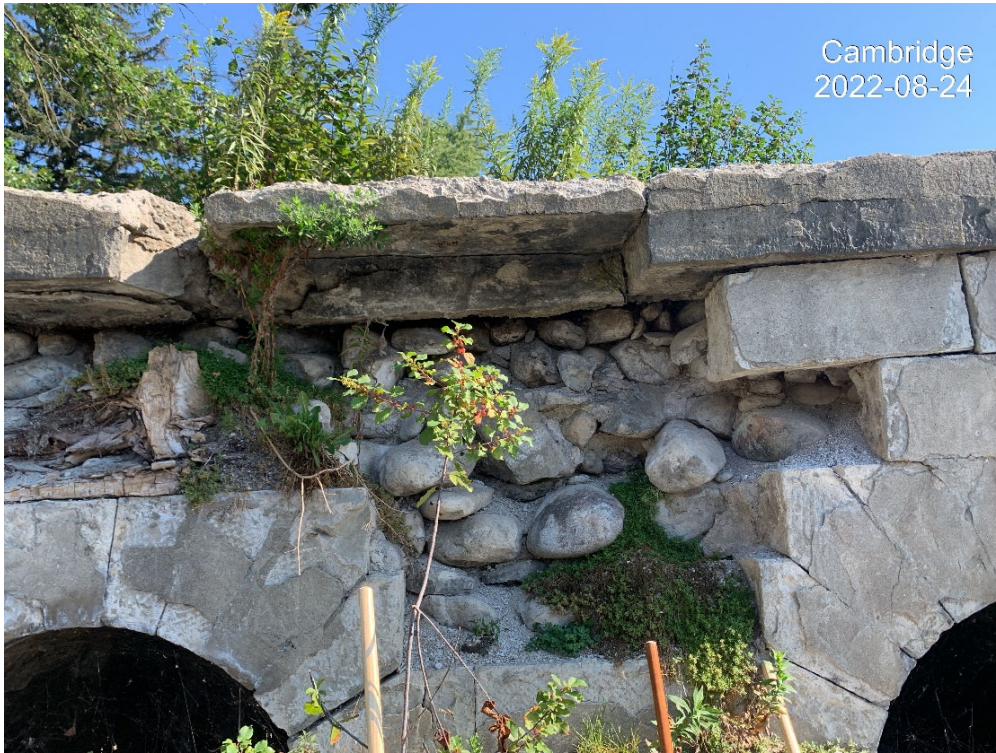
Photo 7 – Vegetation on North Stop Log Structure (1)
