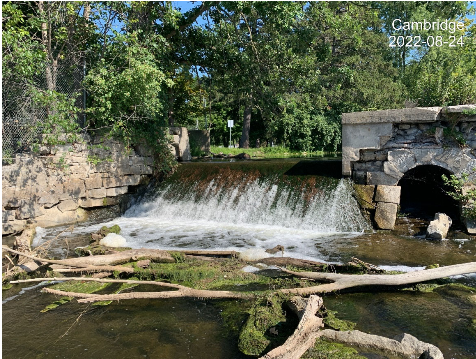
Photo 11 – North Spillway / Erosion along Front Face
