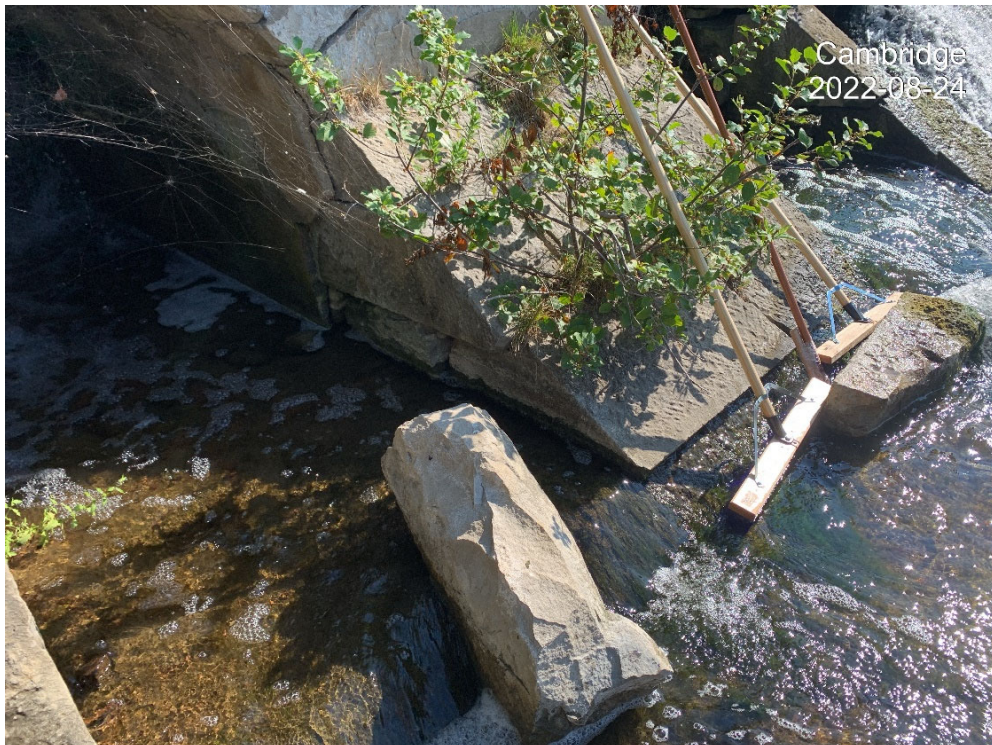
Photo 8 – Vegetation on North Stop Log Structure (2)
