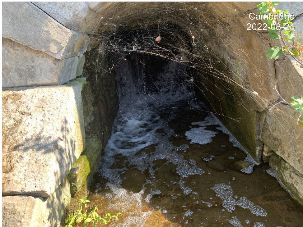
Photo 6 - Leaking Timber Stop Logs on Right Raceway of North Stop Log (Note the Exposed Masonry Blocks)
