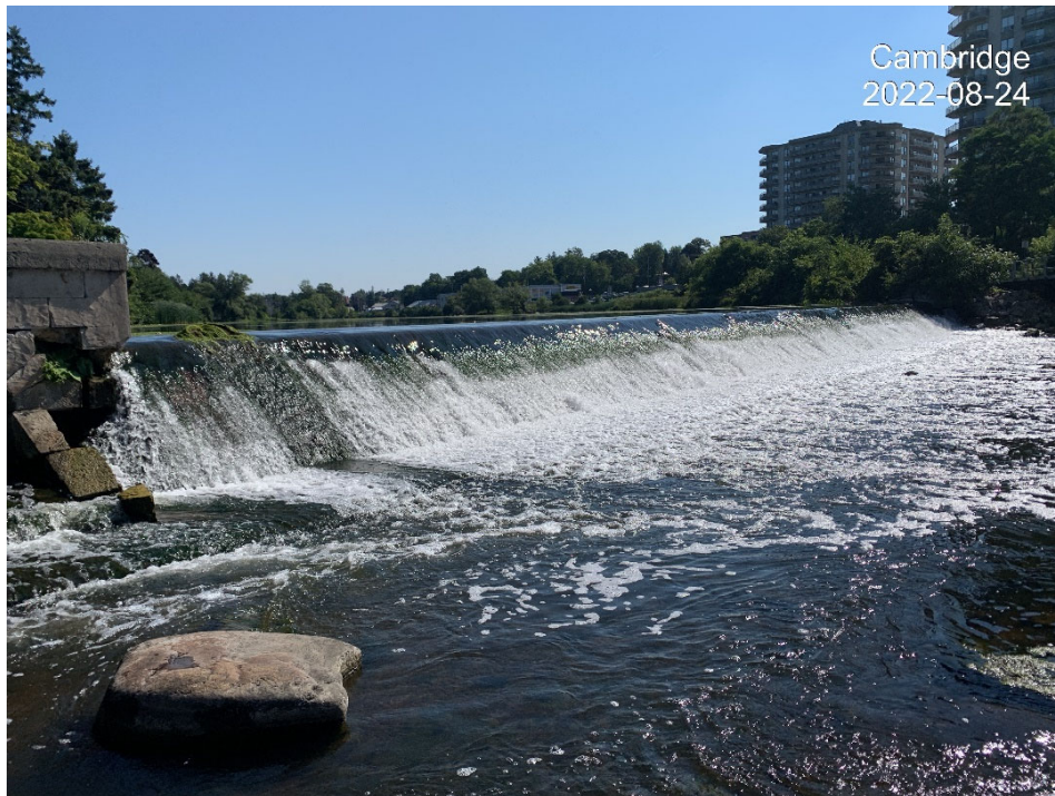
Photo 12 – Central Spillway / Erosion along Front Face
