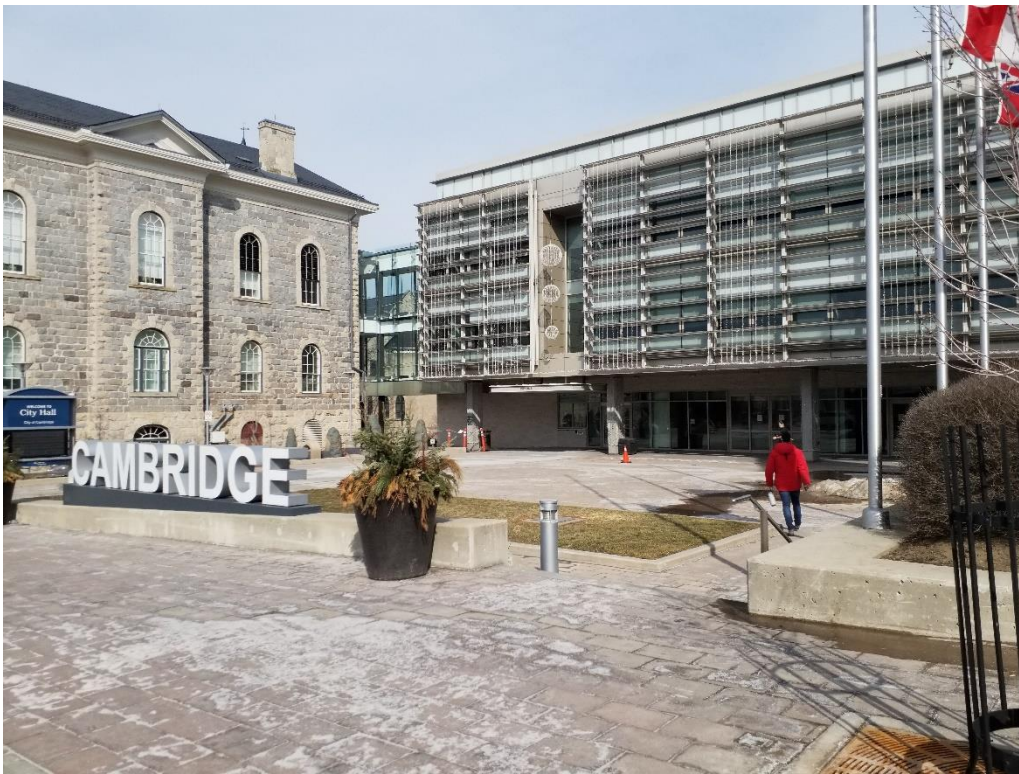
Figure 86: Civic Square with Historic City Hall and Cambridge City Hall (A.S.I. 2021).
