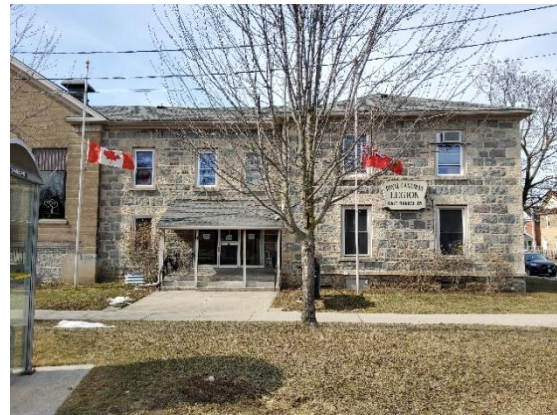
Address: 4 Veteran's Way (Royal Canadian Legion Galt Branch 121) ASI ID: 27 Date of Construction: 1850 Reason for recommendation: This granite house built by local stonemason James Dalgliesh forms part of the collection of colour-matched granite buildings that express the unique vernacular building technique using local stone developed by the Scottish stonemasons who settled in Galt.
