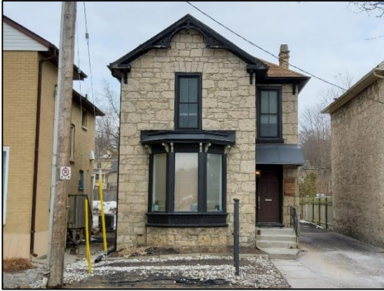
Figure 18: Example of Italianate style at 111 Ainslie Street North.
