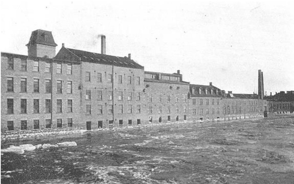
Figure 24: Factories along the Grand River, 1902, not extant (Toronto Public Library).
