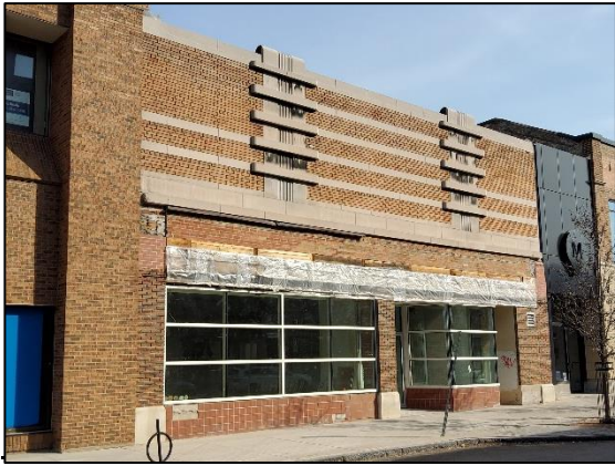
Figure 32: Example of the Art Moderne style at 52-58 Main Street.
