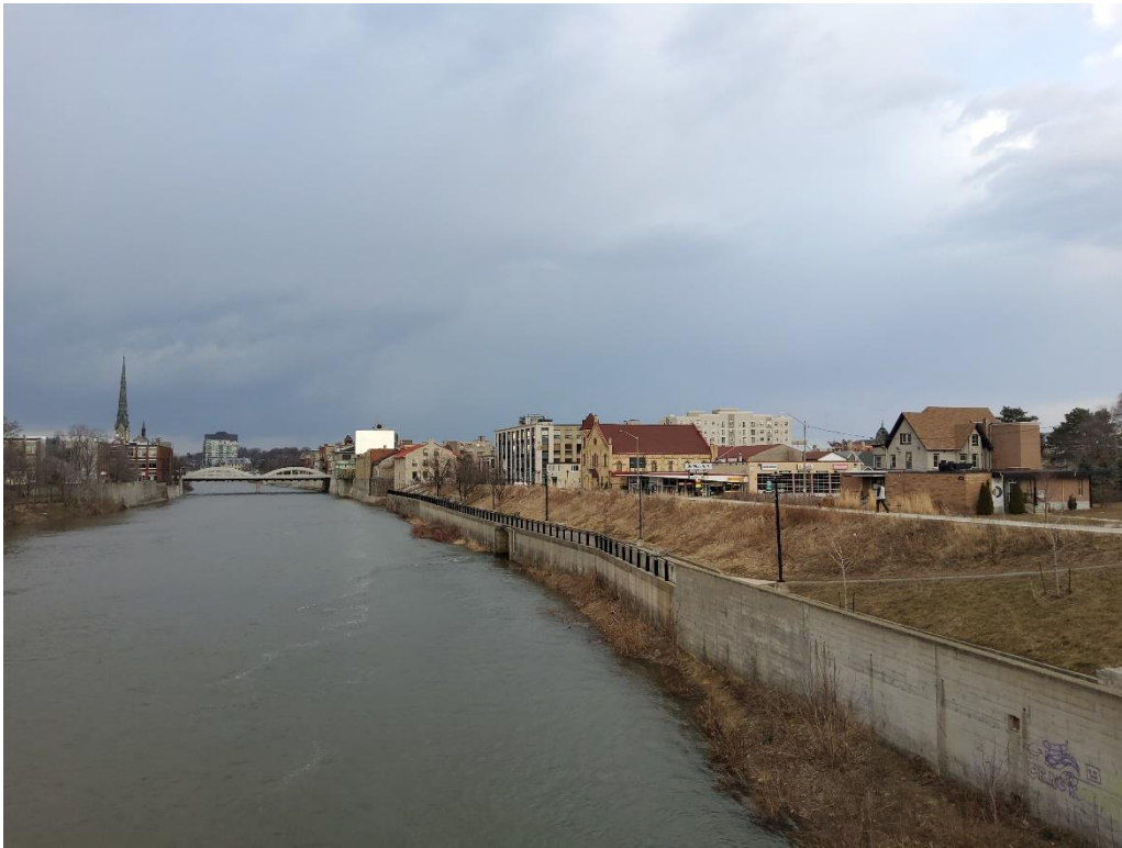
Figure 103: Looking north along Grand River from pedestrian bridge (A.S.I. 2021).
