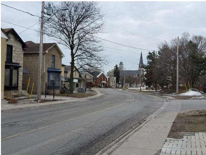
Figure 56: Looking south on Ainslie Street North along curvilinear section resulting from realignment.
