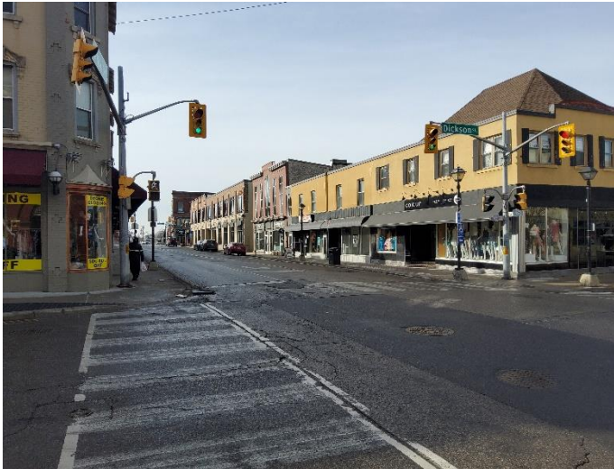
Figure 48: Looking south on Ainslie Street North from its intersection with Dickson Street, showing a continuous commercial context within the streetscape.
