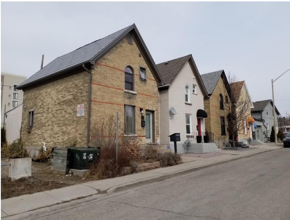
Figure 102: North side of Warnock Street (A.S.I. 2021).
