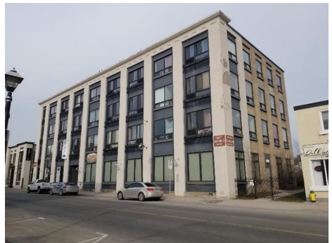
Figure 51: The Galt Knitting Co. Ltd. (Tiger Brand) building with industrial built form and current commercial and residential use.
