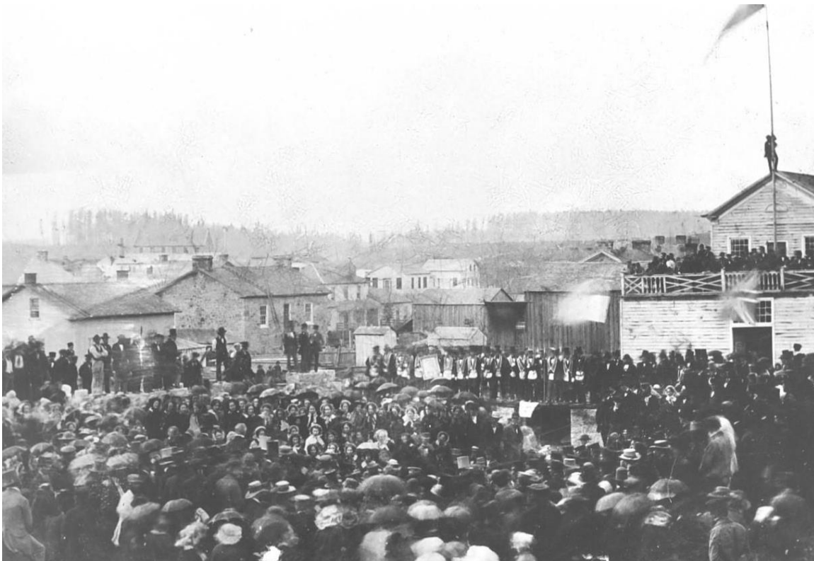
Figure 42: Laying the cornerstone for the Town Hall, Galt, 1857 (City of Cambridge Archives).
