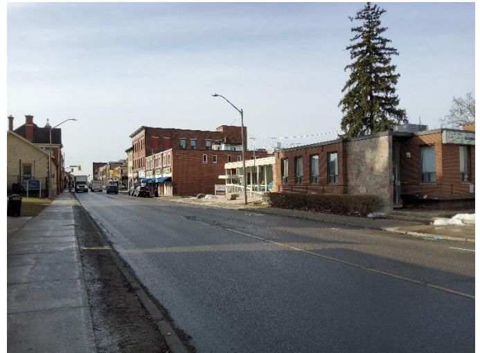
Figure 66: Looking south on Ainslie Street North towards nineteenth- and twentieth-century commercial buildings.
