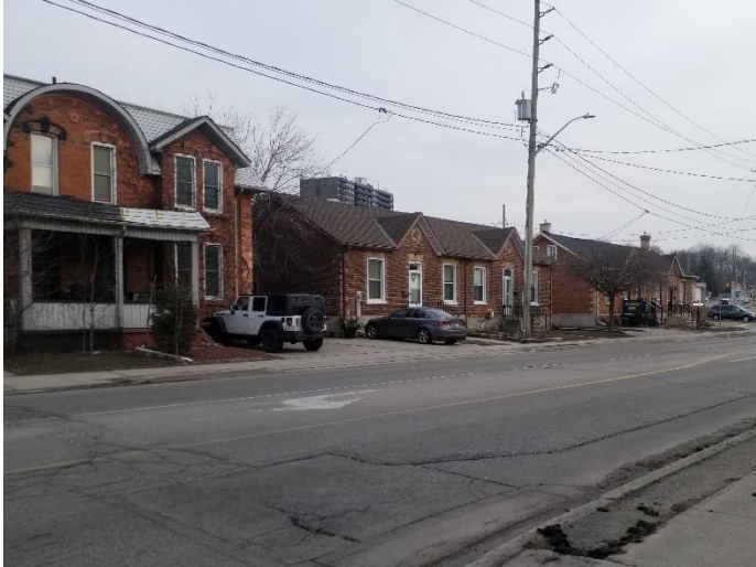
Figure 78: Series of semi-detached houses with red brick cladding on Ainslie Street South.
