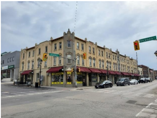
Address: 17-35 Ainslie Street North (Dando Block) ASI ID: 139 Date of Construction: 1881-1882 Reason for recommendation: This unique commercial/mixed-use building is an eclectic example of the Renaissance Revival style and retains some original recessed commercial storefronts on the first storey and is a landmark building at the corner of Ainslie and Dickson Streets.
