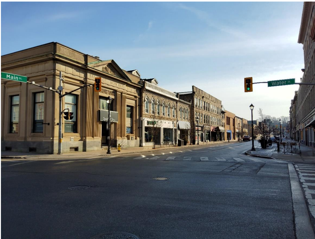
Figure 91: Main Street looking east from Water Street (A.S.I. 2021).
