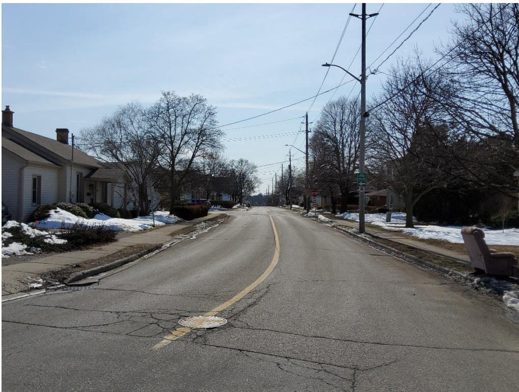
Figure 90: Wellington Street looking south from Kerr Street (A.S.I. 2021).
