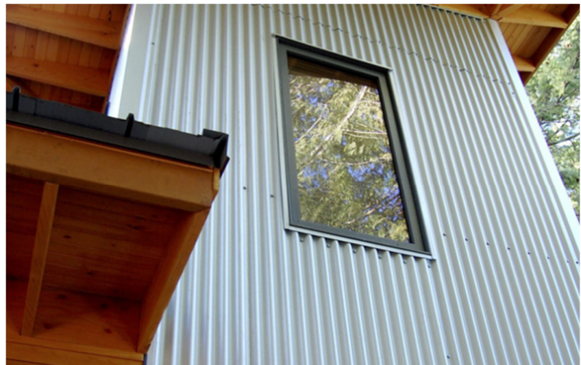
Metal siding at building volume
