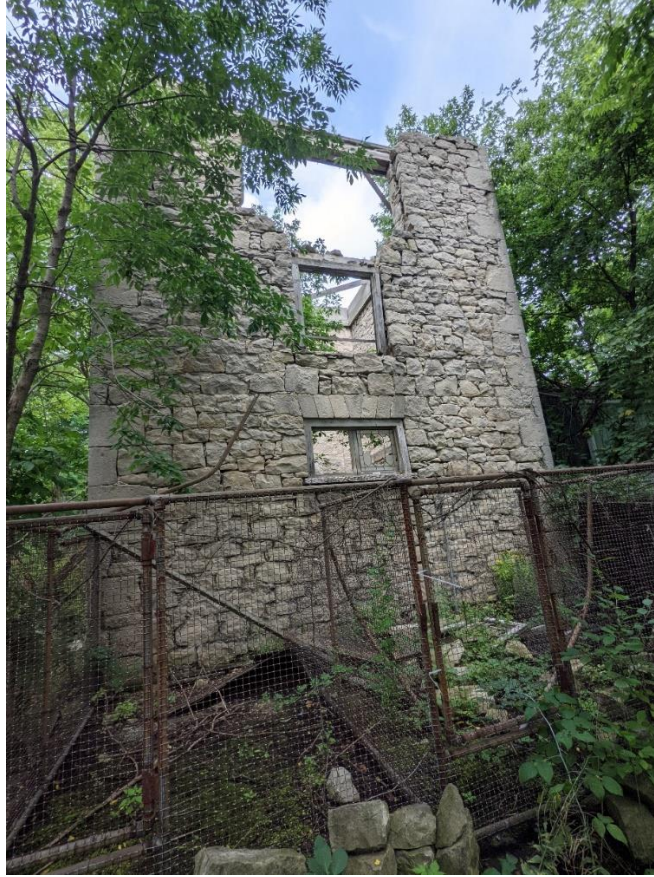
Figure 11: Stone Tower Rear Elevation, August 13, 2021
