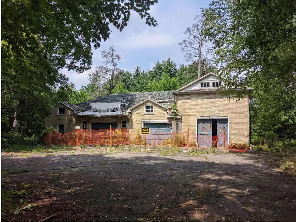
Figure 5: North Garage, August 13 2021
