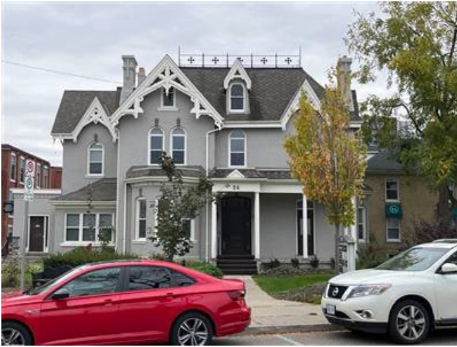
Plate 1: Front Façade (North Elevation) of 24 Queens Square
