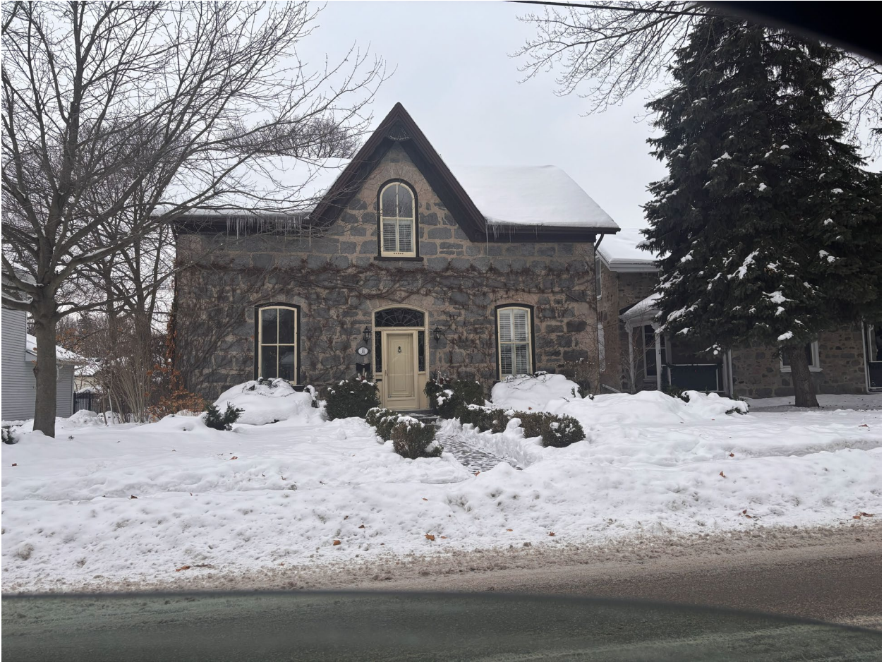
Figure 3 - Picture of the front of 8 Cameron Street taken from the public right of way on December 16, 2025
