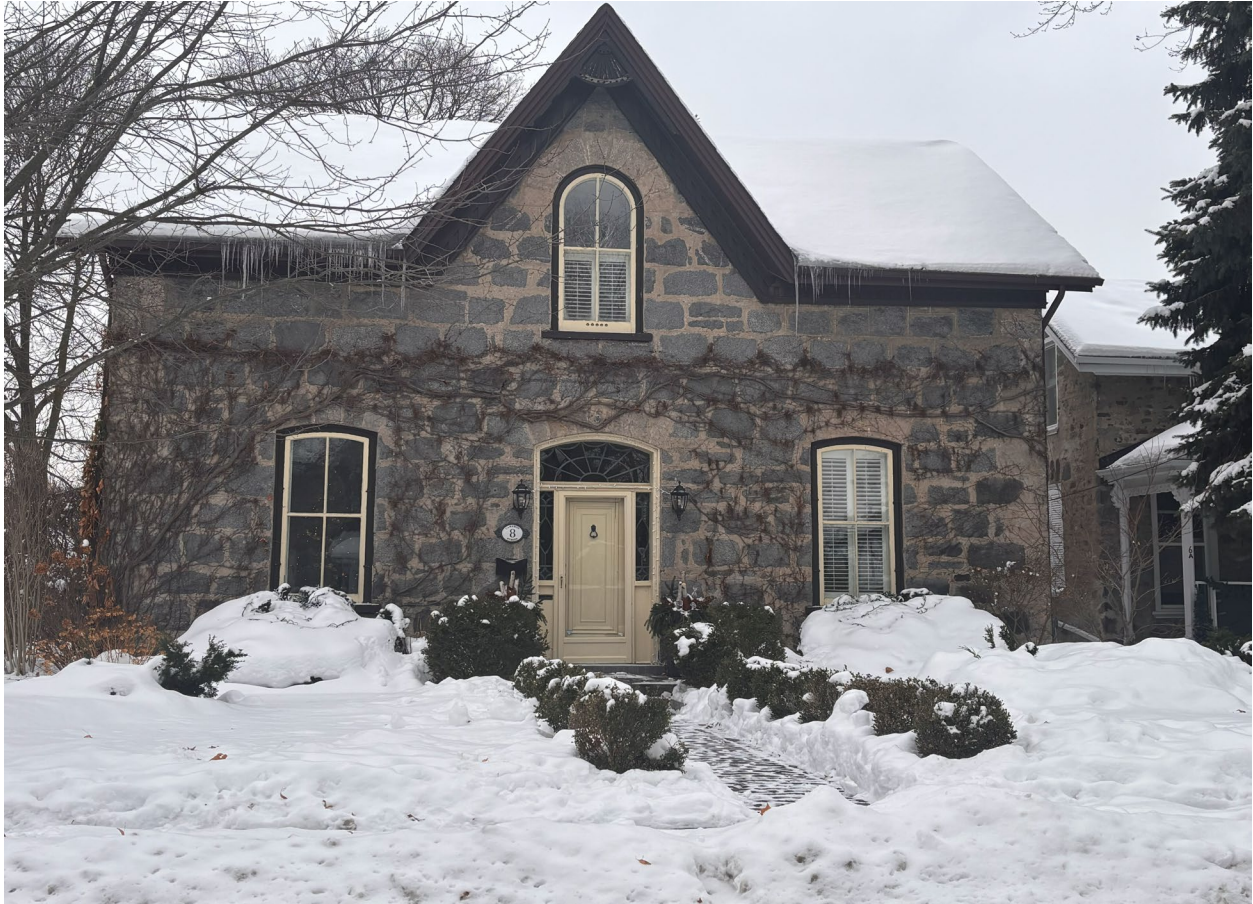
Figure 2 – Picture of the front of 8 Cameron Street taken from the public right of way on December 16, 2025
