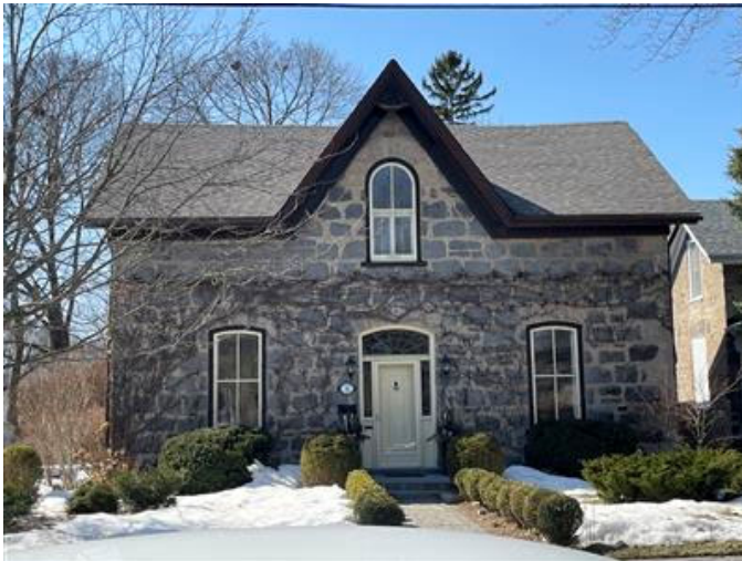
Plate 1: Front Façade (East Elevation) of 8 Cameron Street
