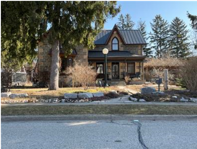
Plate 1: Front Façade (West Elevation) of 77 Lowell Street North
