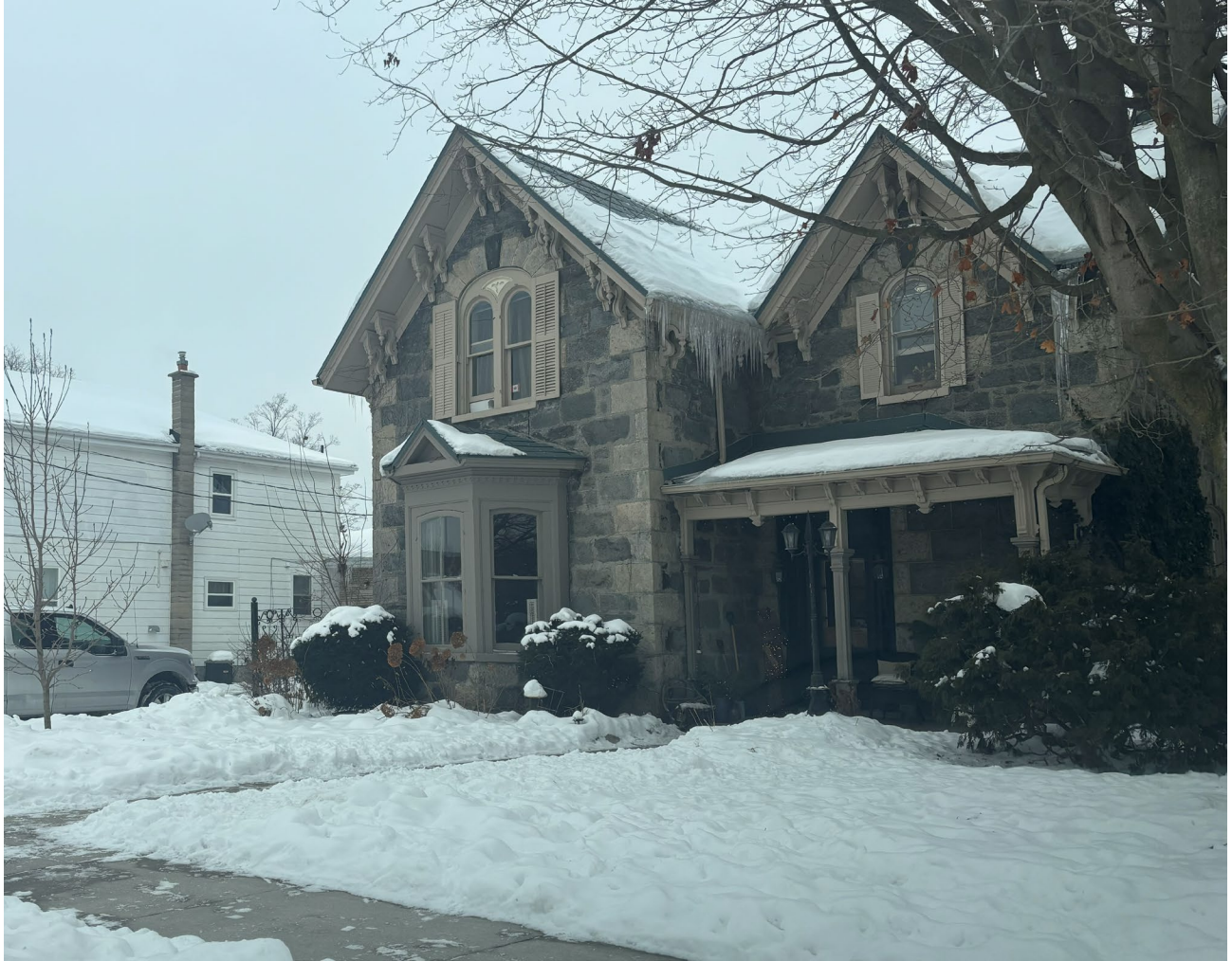
Figure 2 – Picture of 47 Spruce Street taken from the Public Right of Way, December 16, 2025
