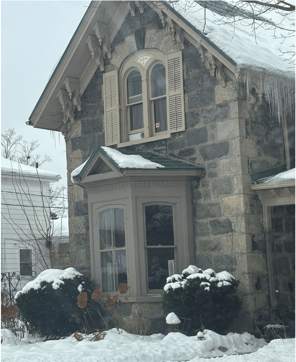
Figure 3 – Picture of the front façade of 47 Spruce Street, showcasing the details of the front, taken from the public right of way on December 16, 2025
