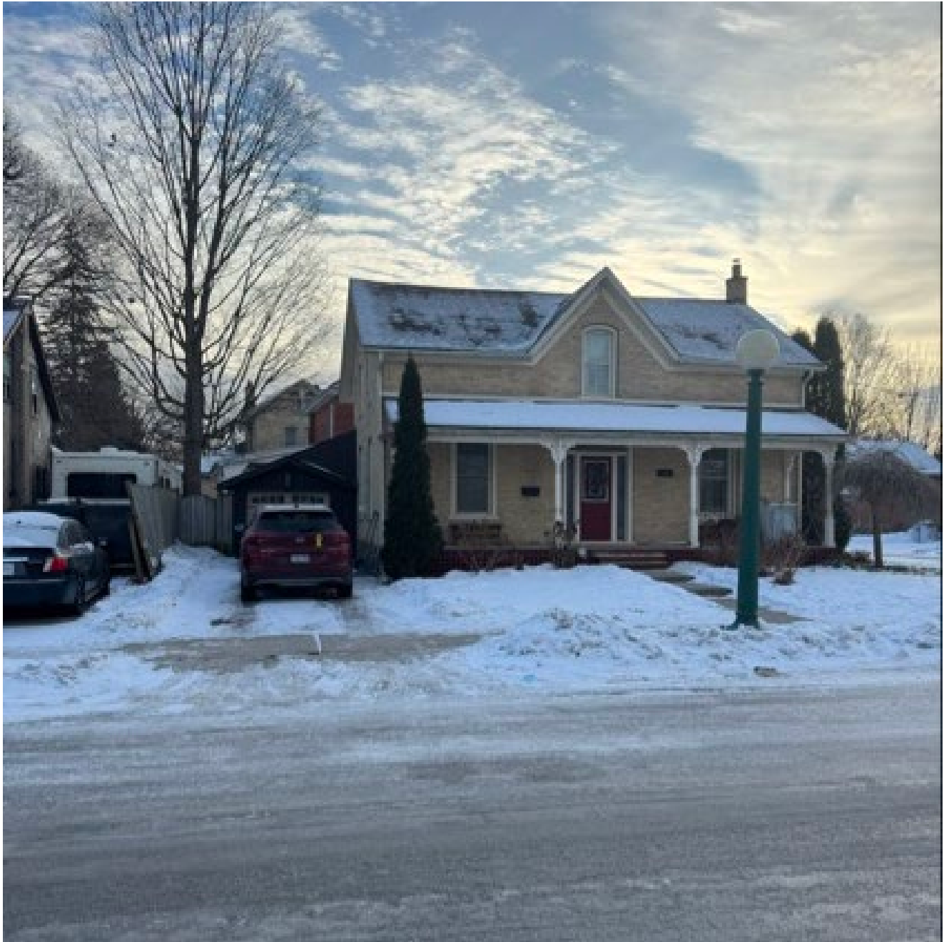
Figure 1 – East (Front) Elevation from Oak Street
