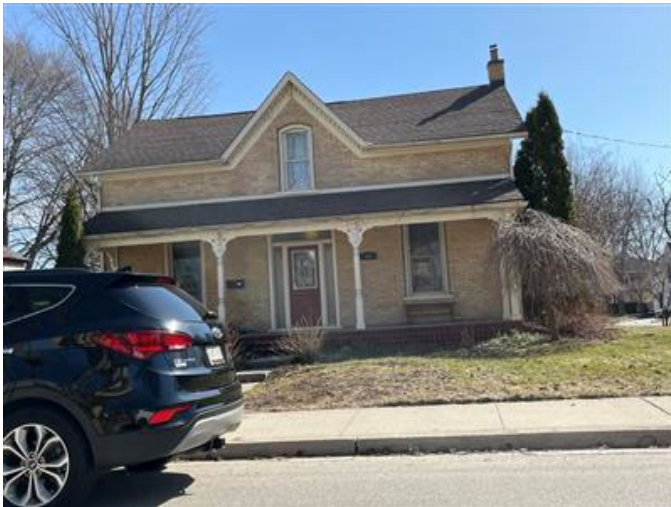
Plate 1: Front Façade (West Elevation) of 39 Oak Street
