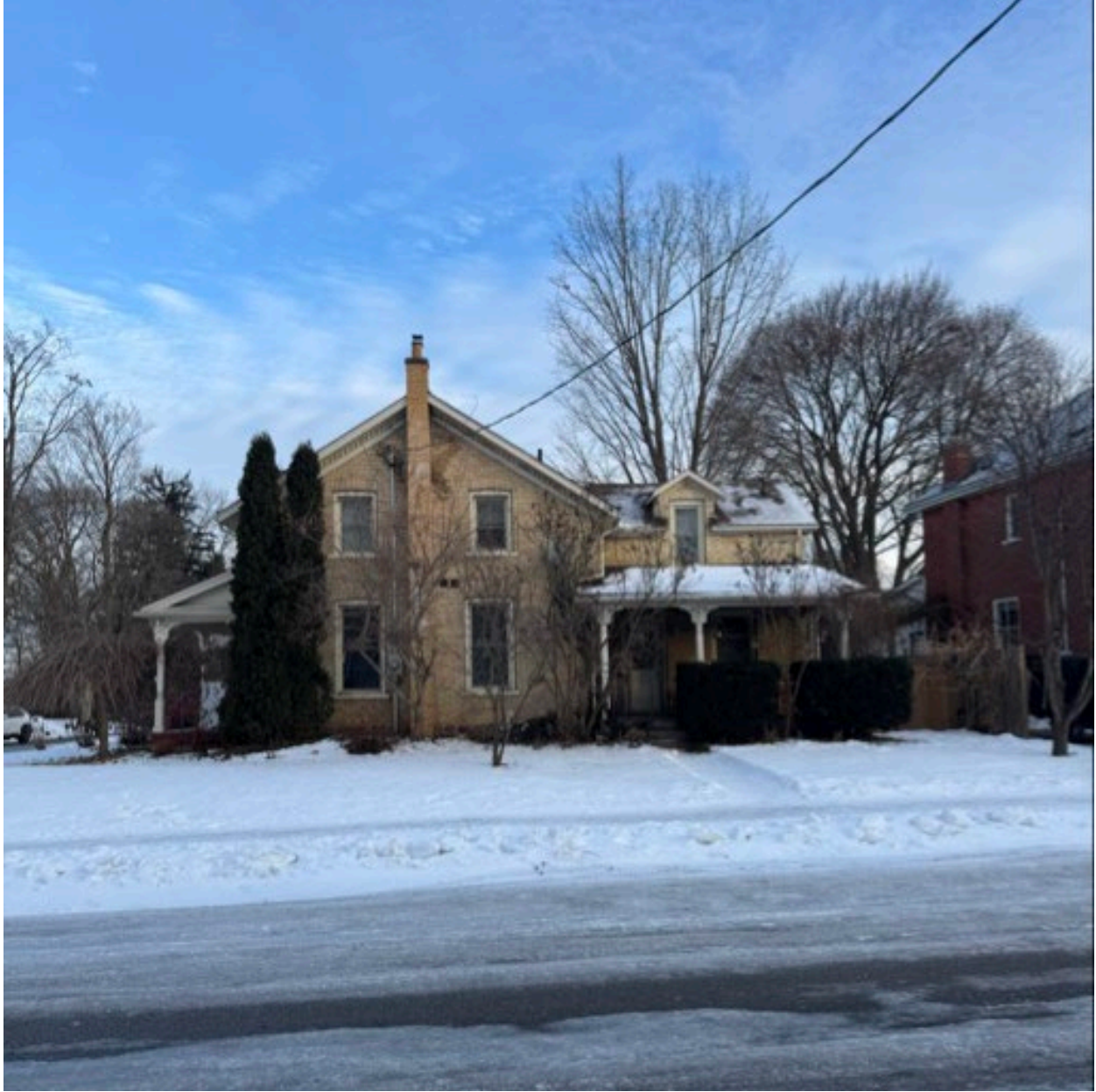
Figure 3 – South- Elevation from Ball Avenue
