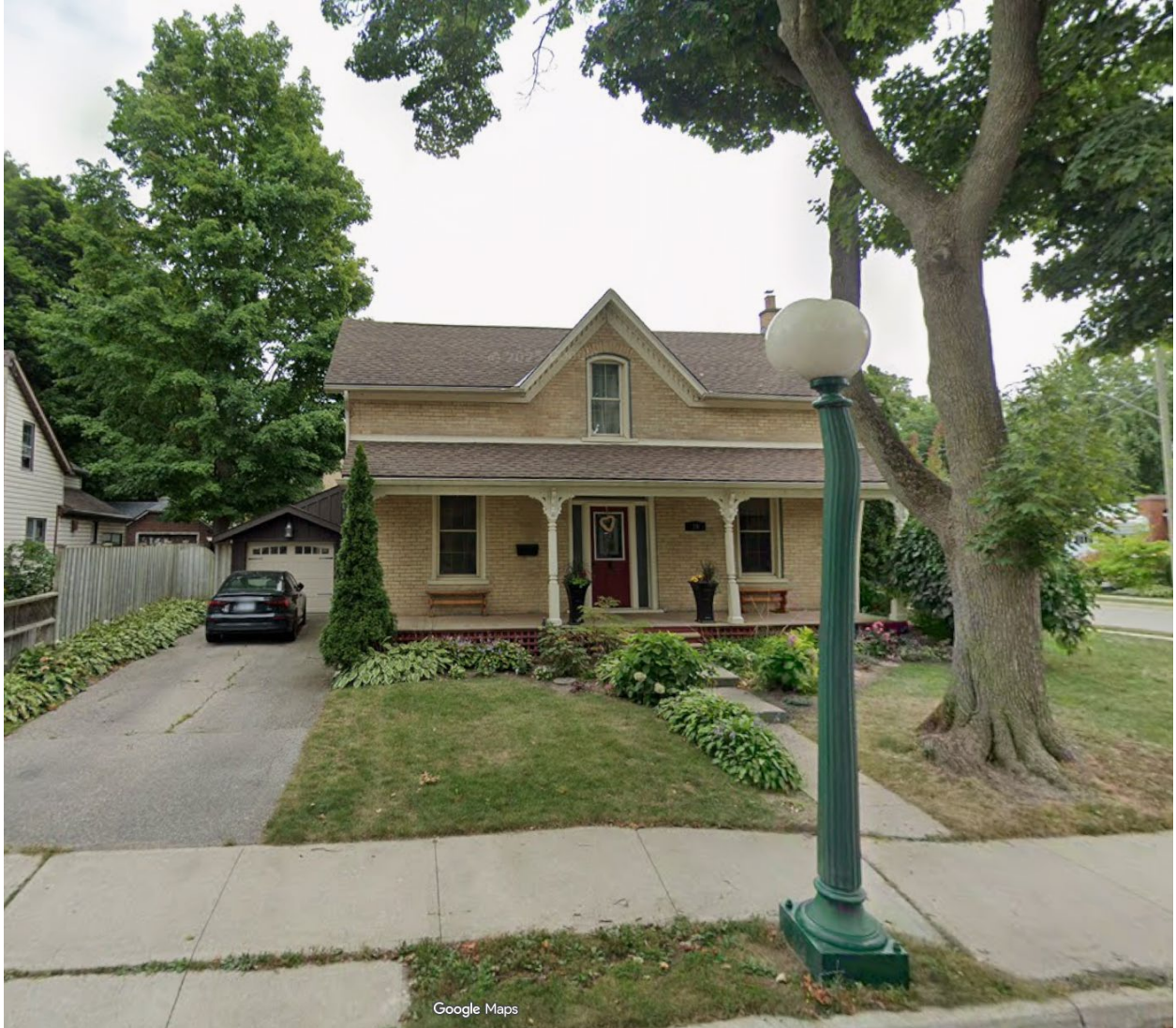
Figure 17 - Google Streetview 39 Oak Street Front Sept 2022
