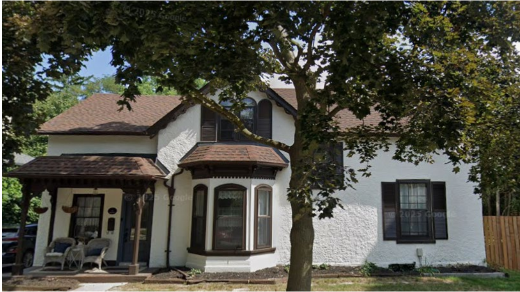
Figure 1: Front Elevation of 11 Kay Street.
