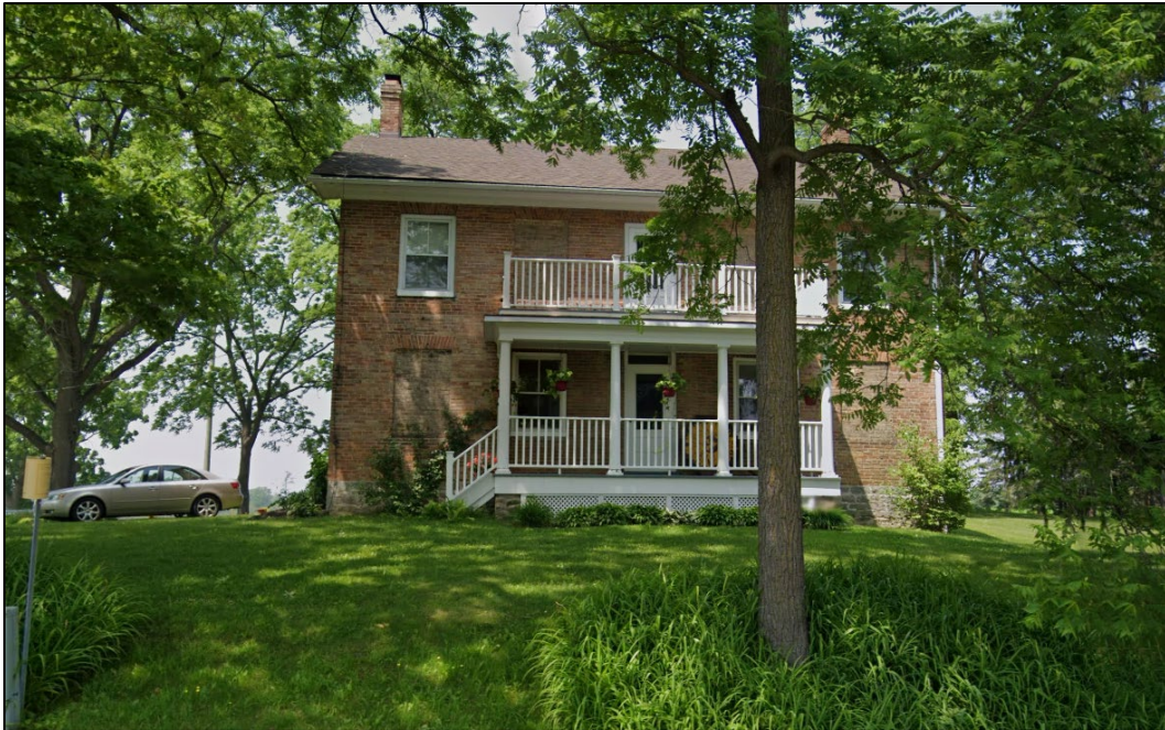
Figure 4: View of the front façade (Google Street View, 2023).
