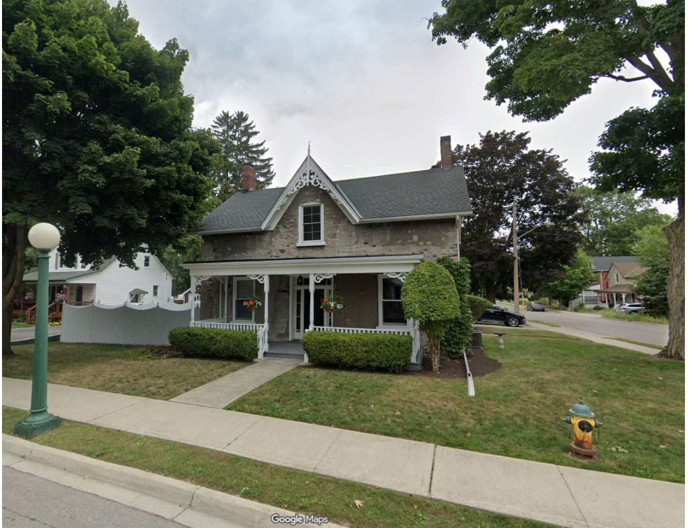
Figure 5 – Google Streetview of 27 Oak Street (West Elevation)
