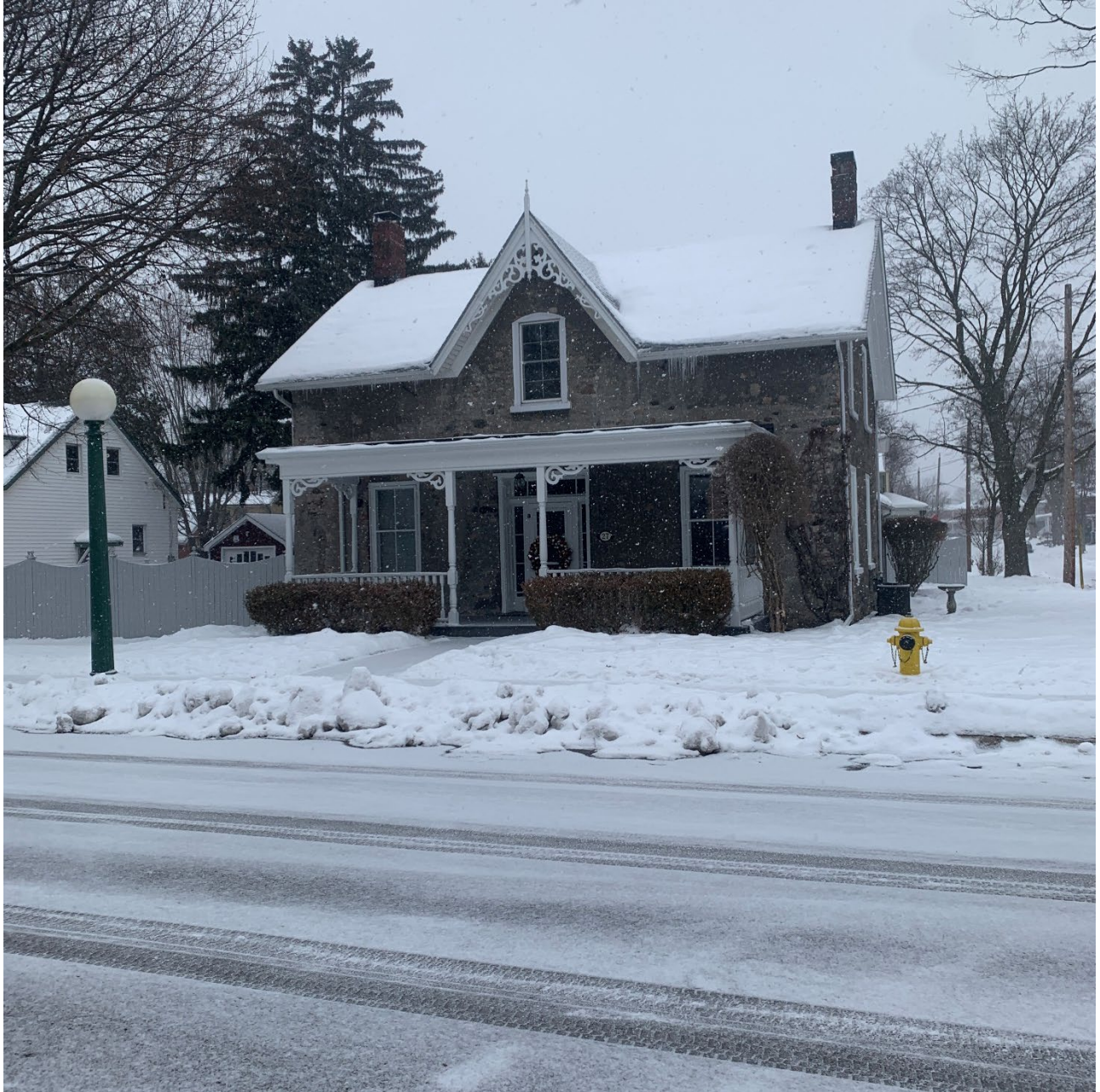
Figure 1 – East (Front) Elevation from Oak Street
