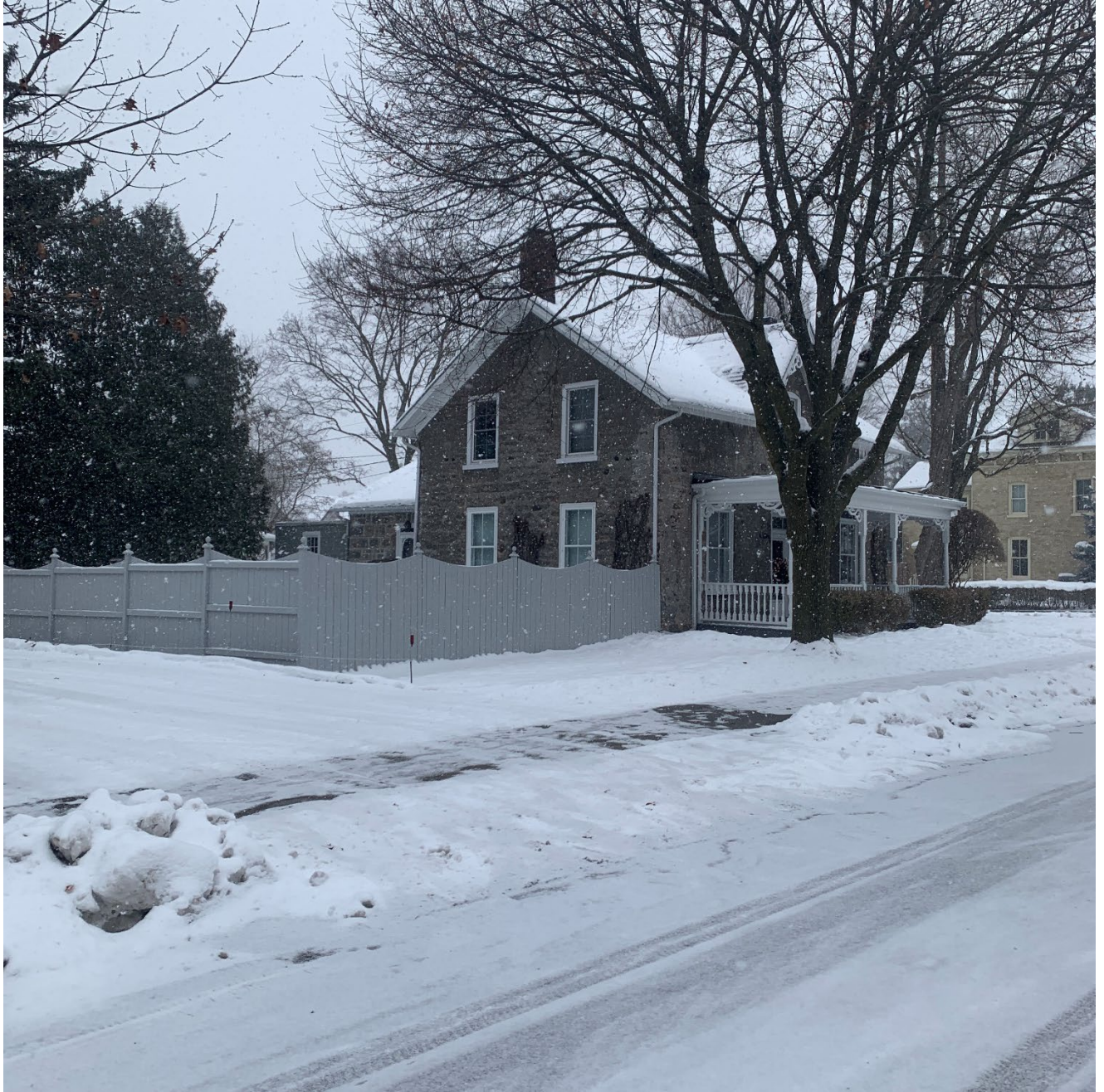
Figure 2 – North – East Elevation from Oak Street
