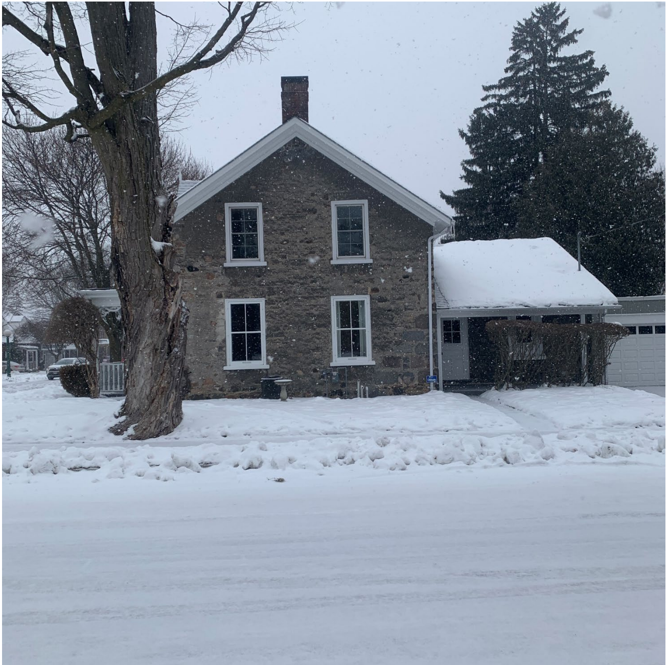
Figure 4 - South Elevation from Rich Avenue
