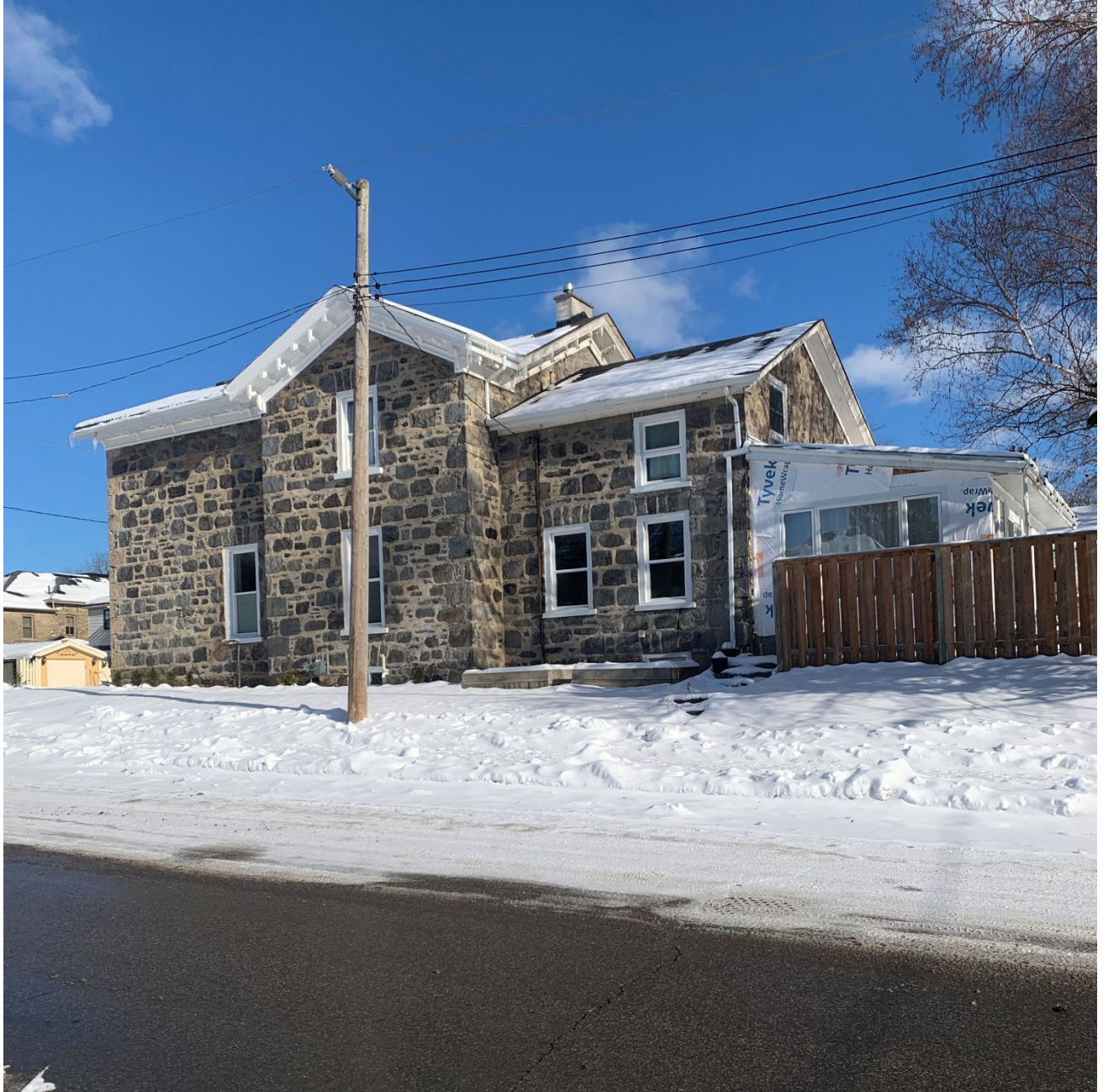
Figure 2 – 59 Bruce Street South- East Elevation from Chisholm Street
