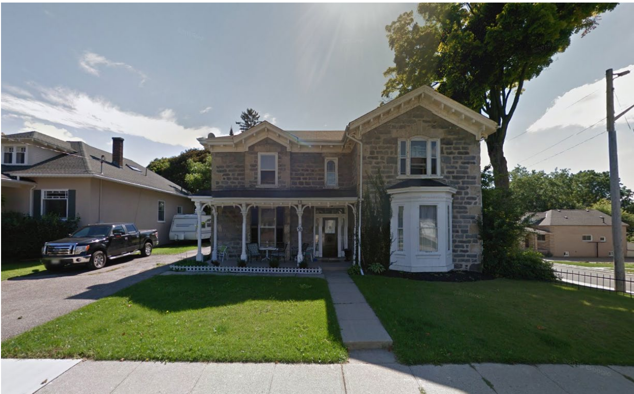
Figure 6 – 59 Bruce Street North Elevation September 2015 Google Street View
