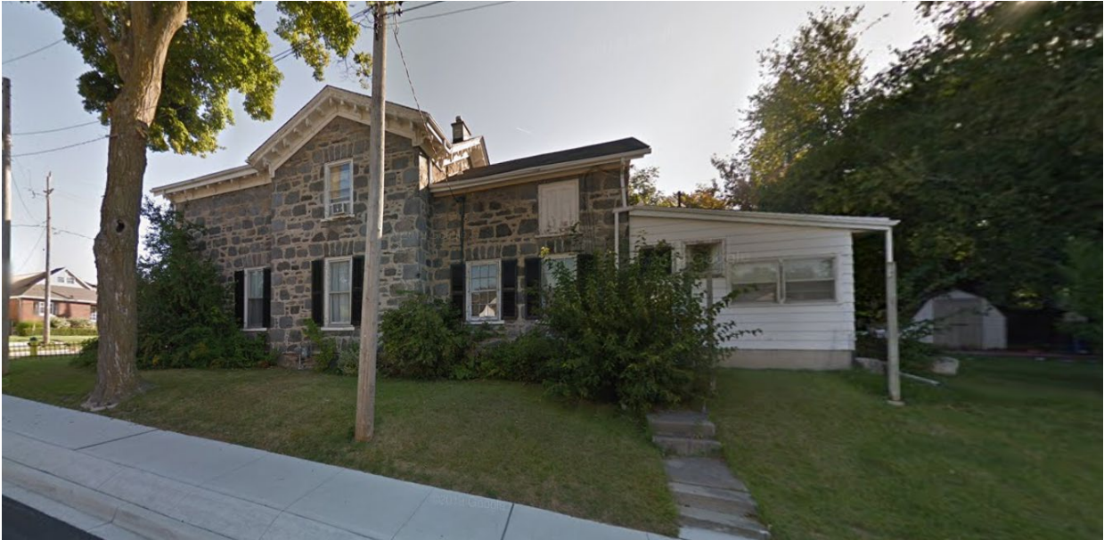
Figure 5 – 59 Bruce Street South East September 2015 Google Street View
