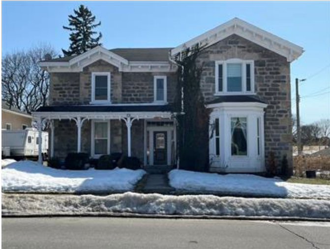
Plate 1: Front Façade (North Elevation) of 59 Bruce Street
