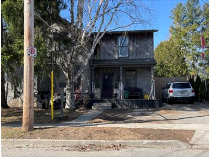
Plate 1: Front Façade (East Elevation) of 78 Chalmers Street
