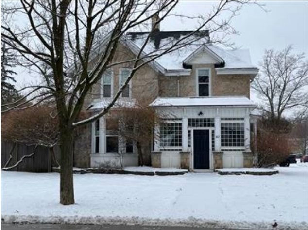
Plate 1: Front Façade (east elevation) of 82 Glenmorris Street
