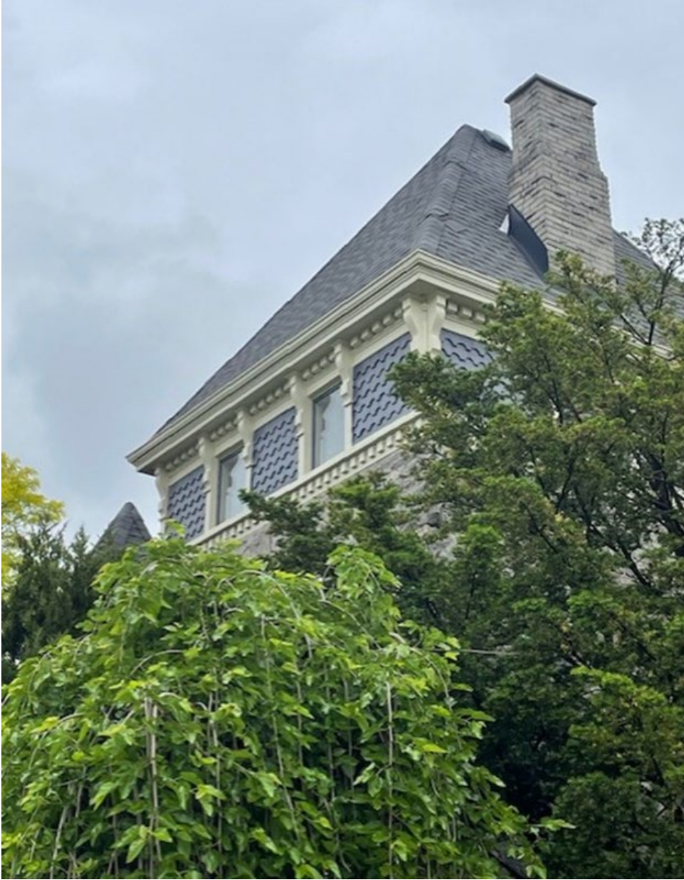
Figure 3: Upper cornice and attic-level windows (Scott Abbott, June 2025).
