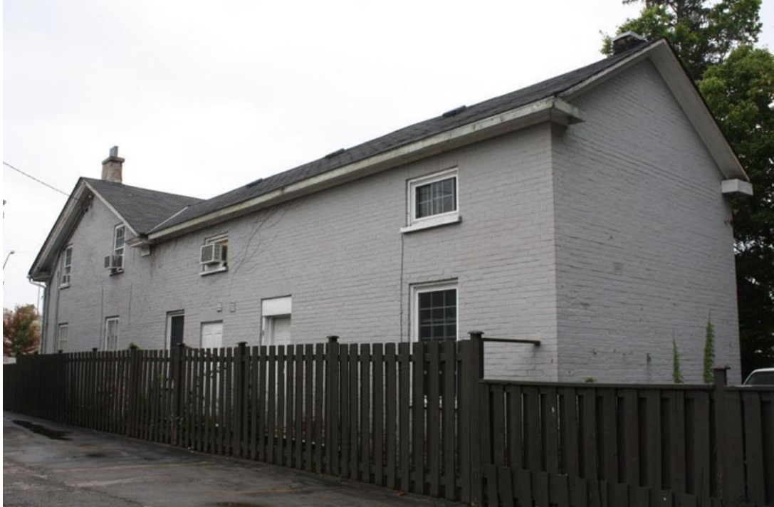
Figure 3: Photograph of the north (rear) elevation, illustrating the long gable-roofed tail extending behind the main block.
