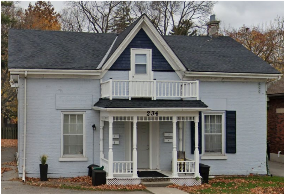
Figure 1: Photograph of the south (front) facade of 234 King Street East, showing the painted brick exterior, centre gable and two-storey porch (Google Maps street view, November 2024).
