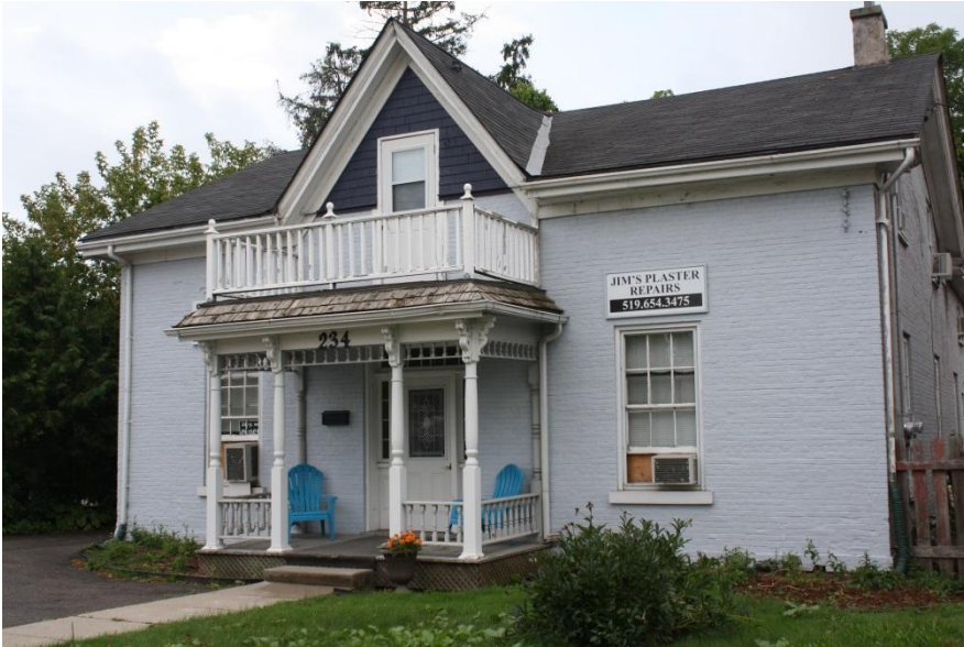
Figure 1. Front elevation of 234 King Street East (AB, 2014)
