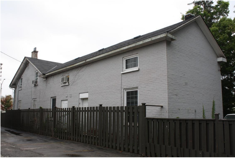
Figure 3. Northern elevation (rear) of 234 King Street East (AB, 2014)
