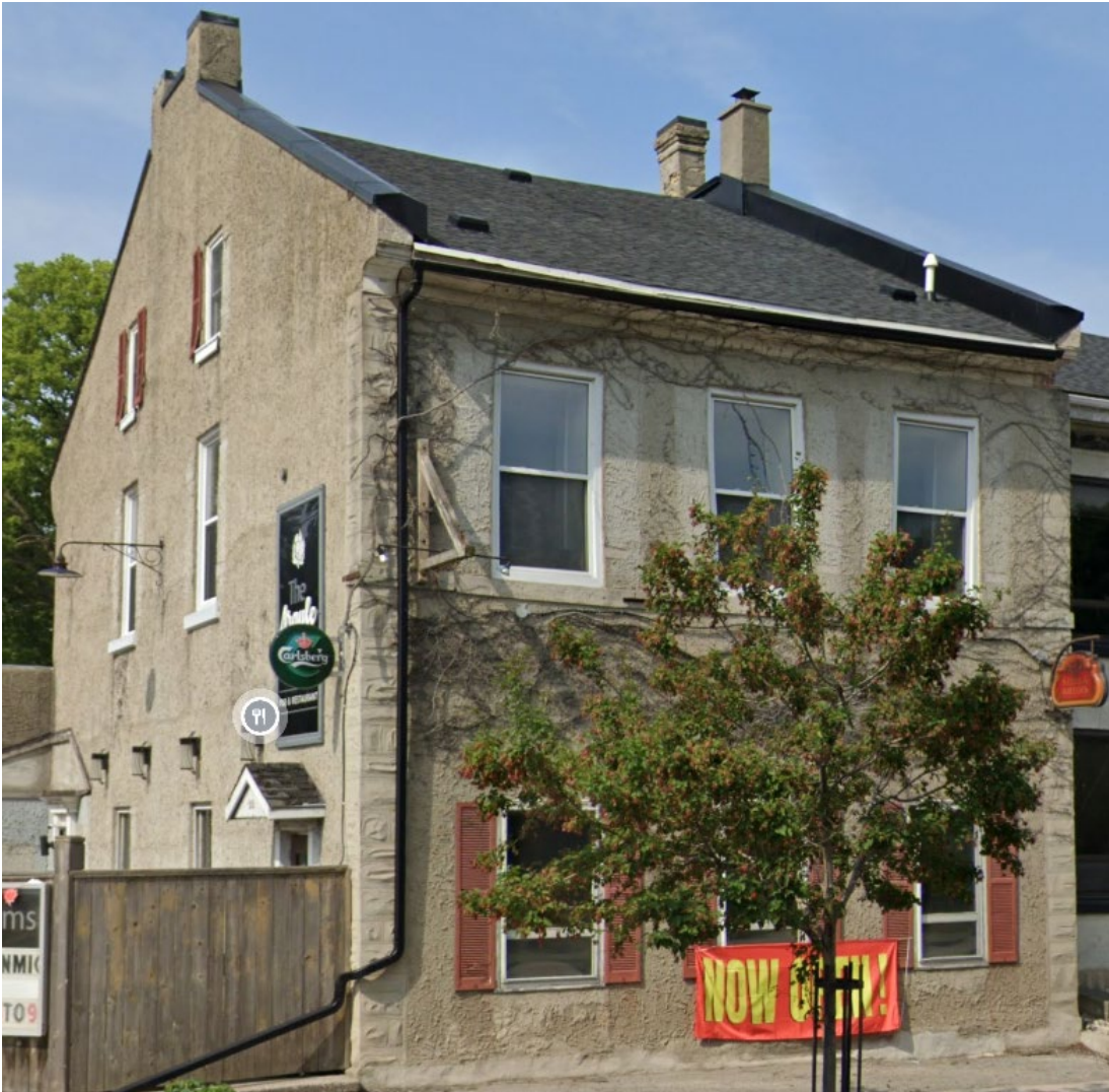
Figure 1: Front Elevation of 210 King Street East (Google Maps, 2023)
