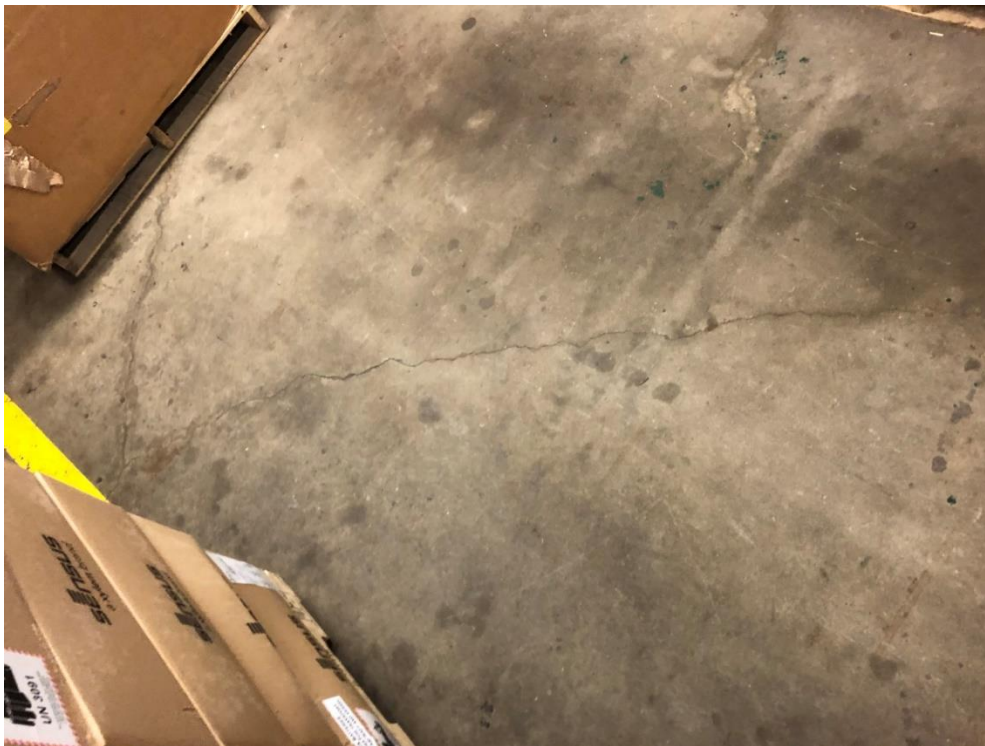
Photo 8 – View of the typical condition of the interior concrete slab-on-grade
