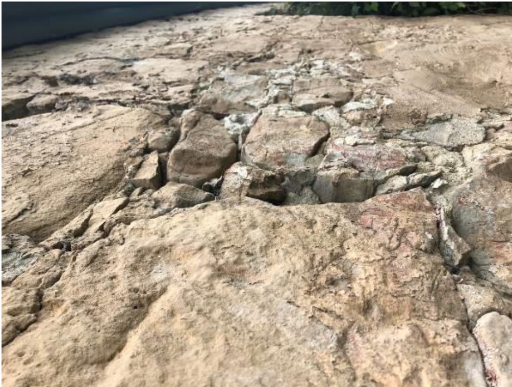
Photo 7 – View of typical stone rubble masonry deterioration
