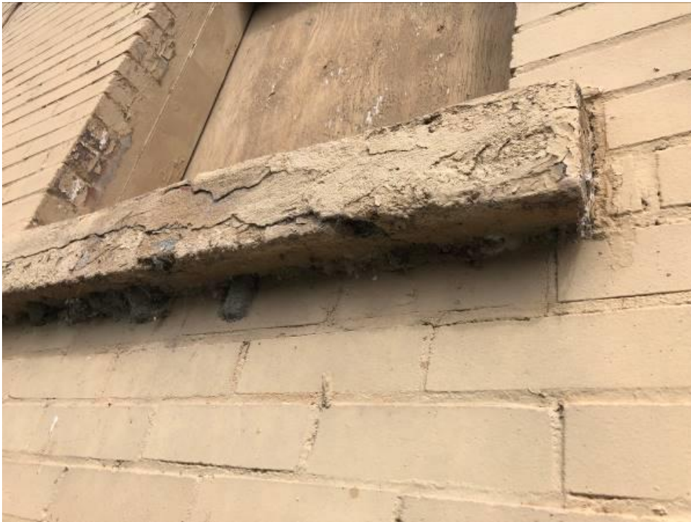
Photo 17 – View of the window sill deterioration on the south elevation of building Section S.4
