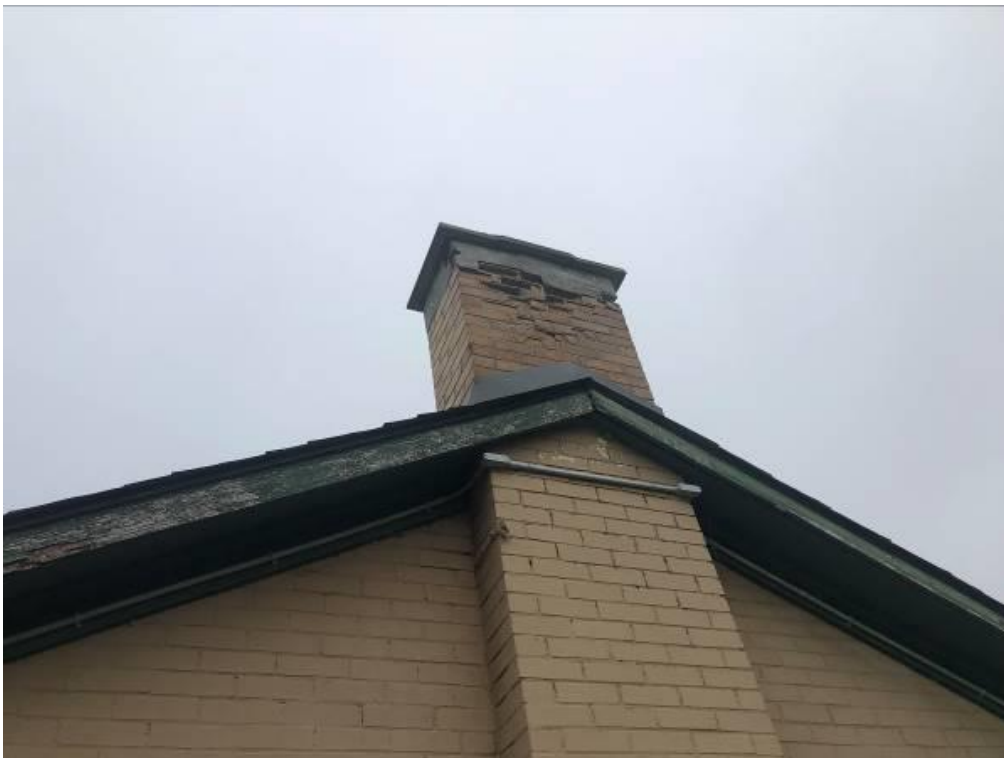
Photo 16 – View of brick masonry spalling at the chimney on the east elevation of building Section S.4
