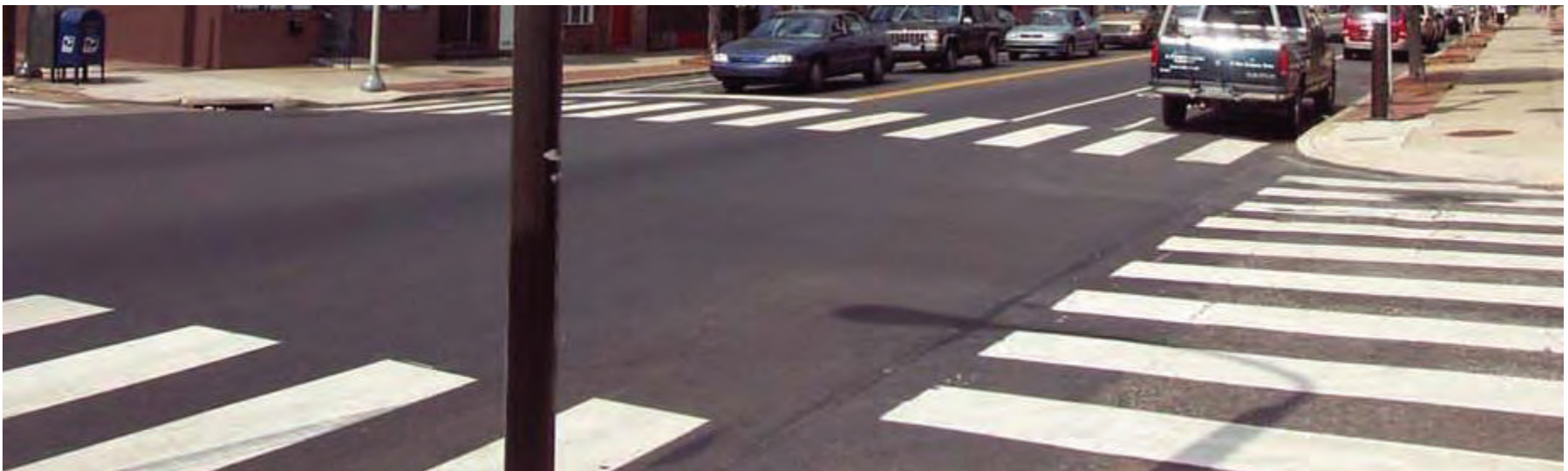
EXAMPLE: THERMOPLASTIC PEDESTRIAN CROSSING
