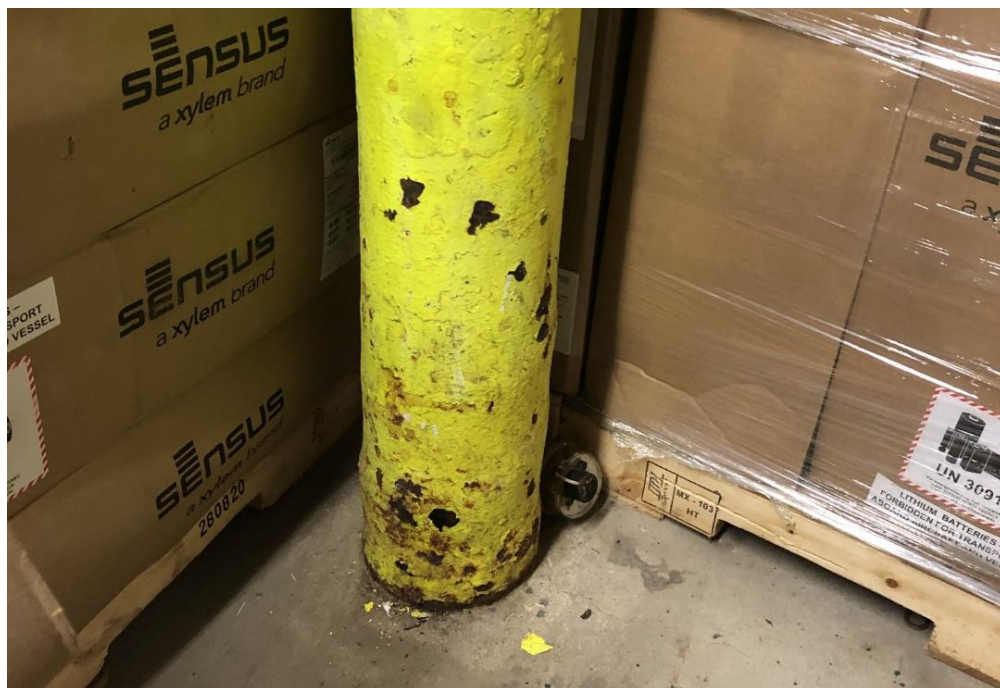
Photo 6 – View of typical localized steel corrosion at base of interior support column located in Section S.1.
