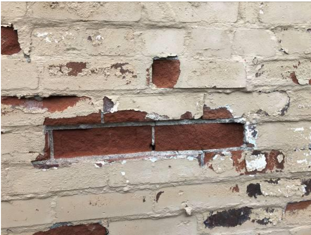
Photo 10 – View of typical localized spalling of the perimeter brick masonry walls.
