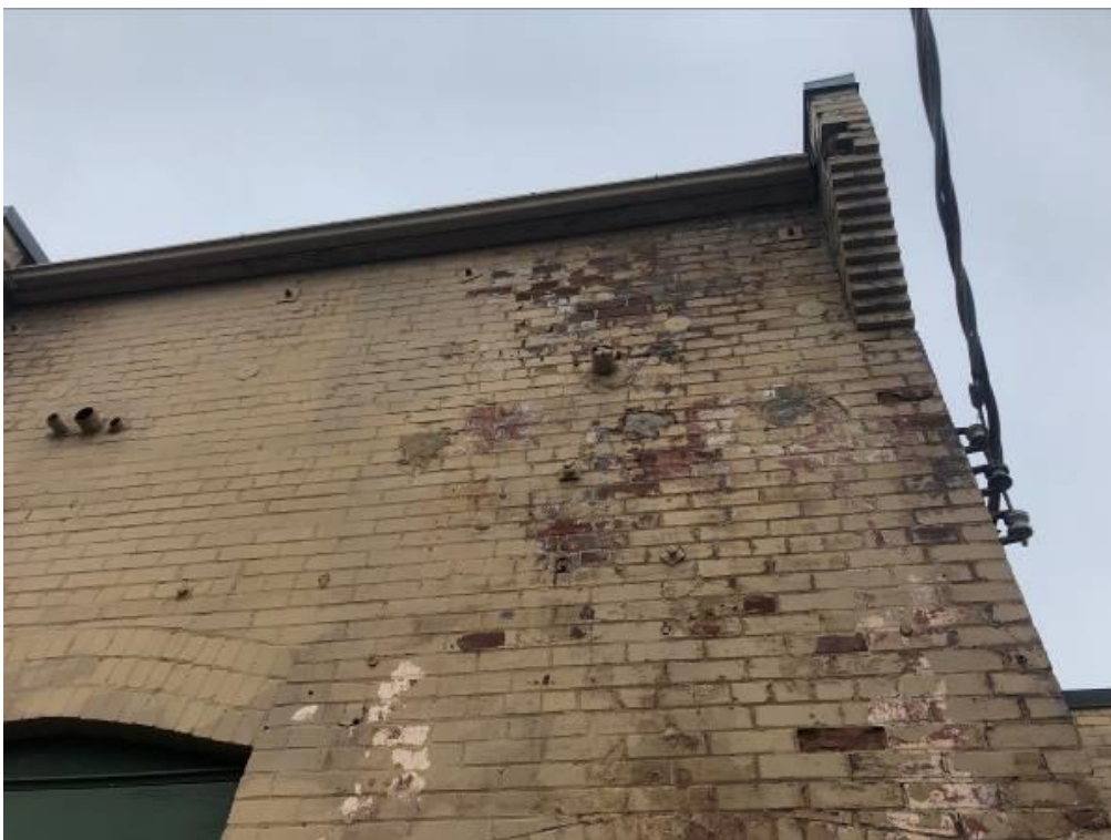
Photo 14 – View of brick masonry wall and corbel deterioration at the north elevation of building Section S.3
