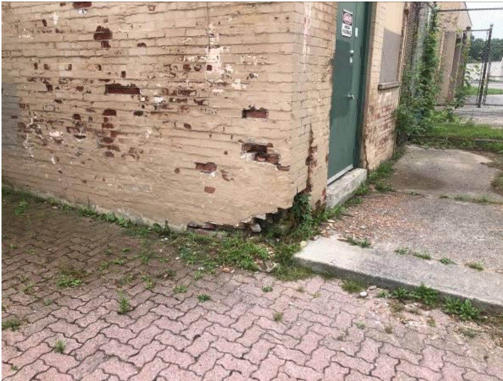
Photo 13 – View of the brick masonry deterioration at grade at the northeast corner of building Section S.3
