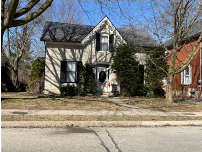
Plate 1: Front Façade (East Elevation) of 26 Oak Street
