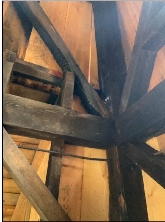
Photograph 6: Charring damage
