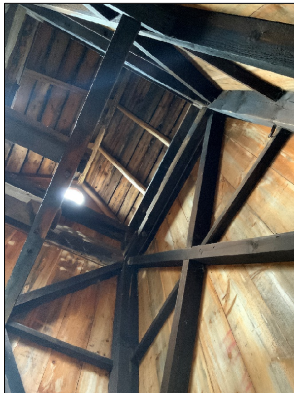
Photograph 4: Upper roof framing
