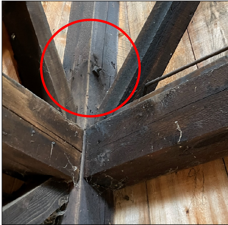
Photograph 2: Connection between upper and lower column sections
