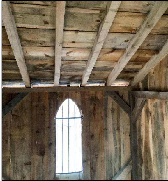
Photograph 5: Lean-to framing (typical)
