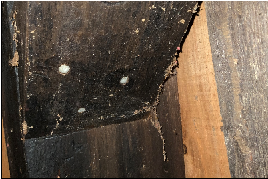
Photograph 3: Connection of diagonal brace to column (south elevation)
