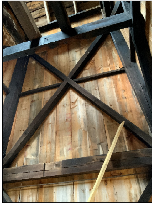
Photograph 1: Partial interior elevation
