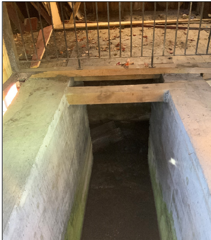
Photograph 9: Water intake foundation walls
