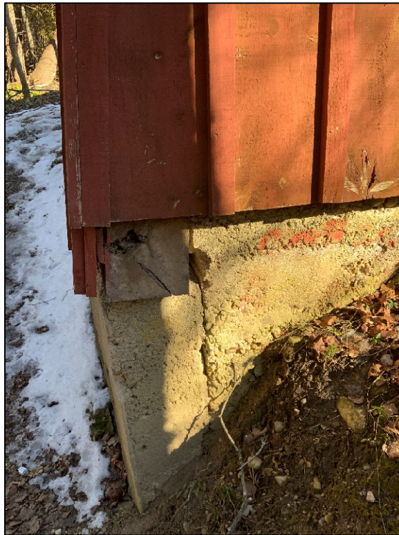
Photograph 7: Exposed foundation wall at northwest corner
