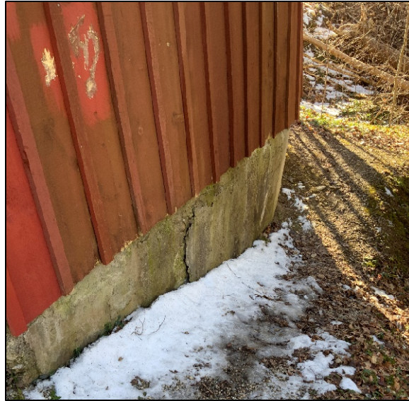
Photograph 8: North foundation wall
