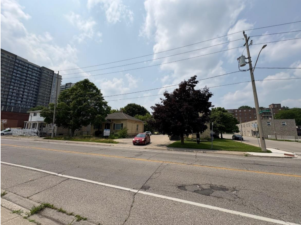
Figure 1 - View of the Subject Lands from the east side of Grand Ave S.
