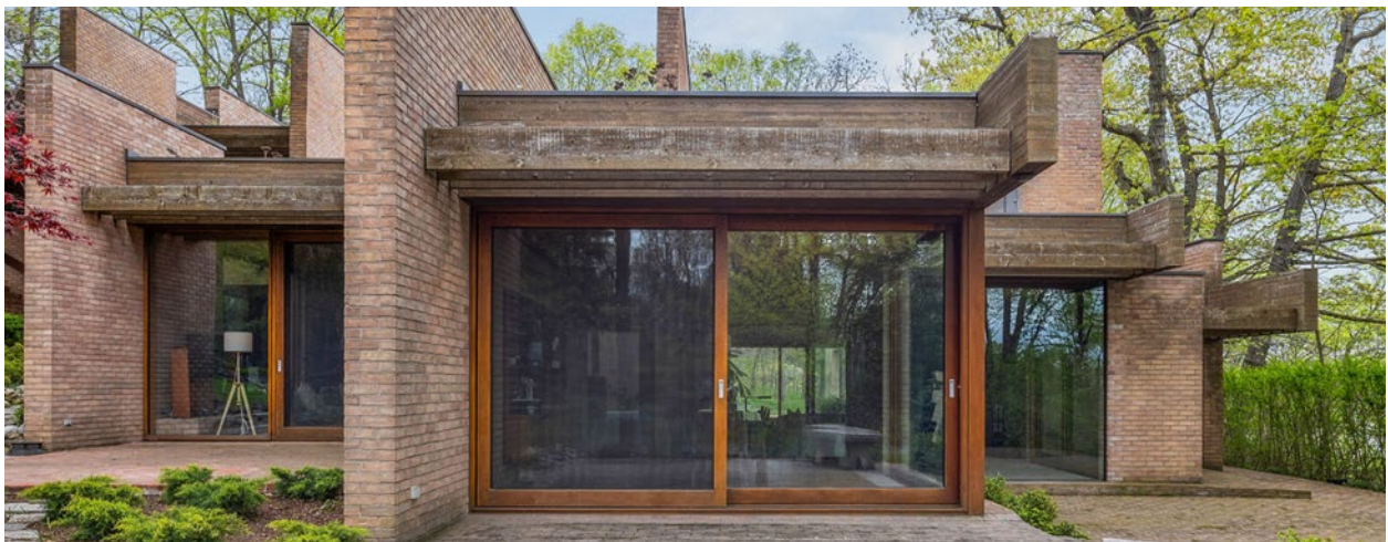
Figure 7: Deep-set glazing and treetop surroundings reflecting Erickson's emphasis on indoor-outdoor continuity (Sotheby's Realty of Canada).
