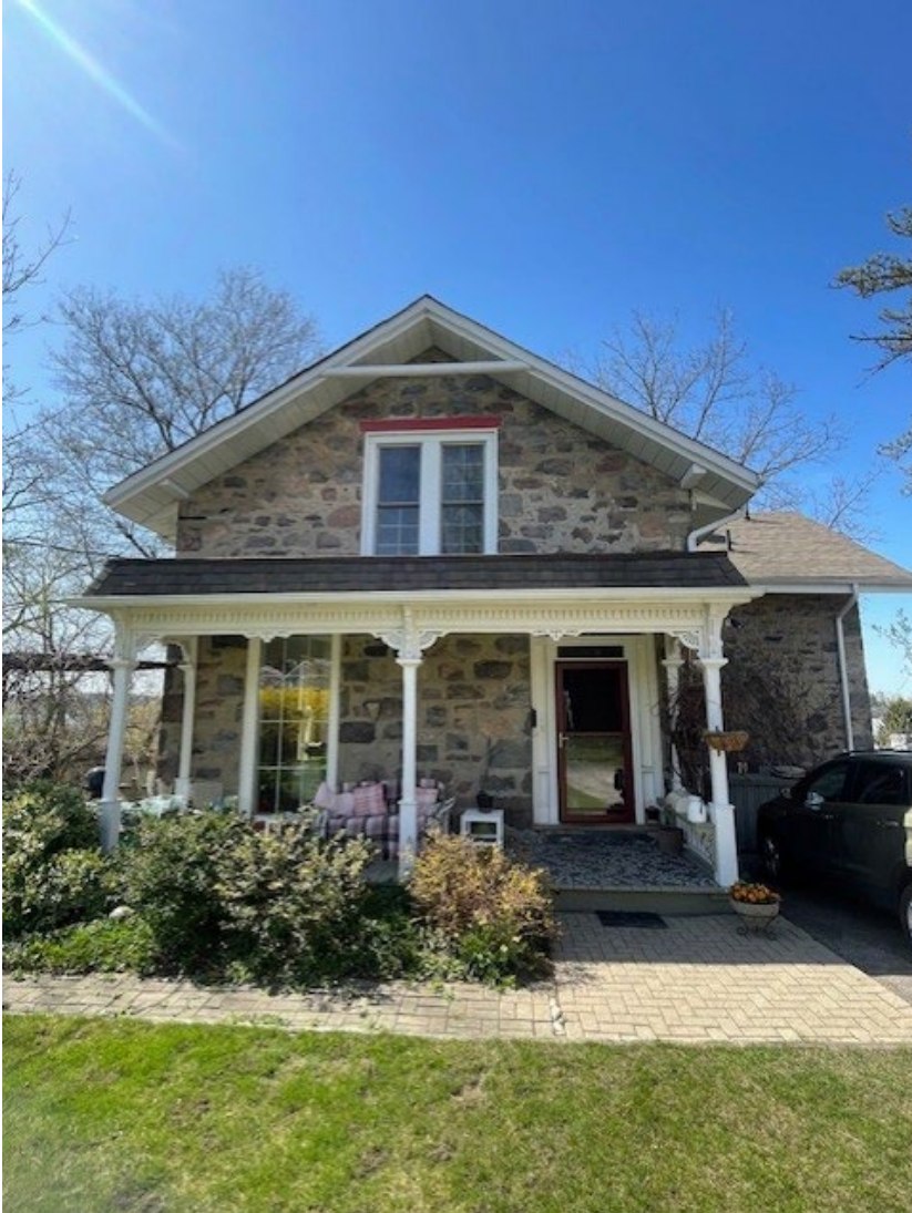
Figure 1: Front façade of 70 Oak Street (Scott Abbott, April 2025)
