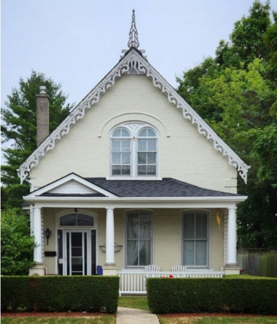
Figure 1: Front façade of 119 Wellington Street (Cambridge Today, 2025)
