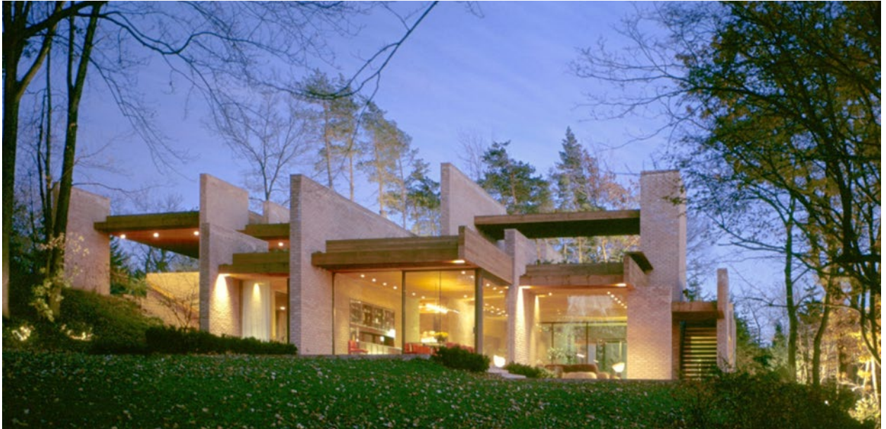
Figure 1: Garden-side Elevation of 194 Blue Heron Ridge (Arthur Erickson Foundation)
