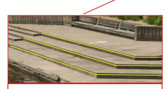
Top three risers to have a ¾ inch channel cut into front face of the riser. This will allow for LED IP68 tape light to be housed in a recessed channel. Power and data to be fed from new panel.
