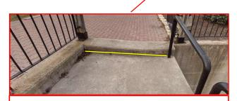
Use small space/groove under steps to house LED RGBW strip. Power to be supplied from cabinet located on the street.
