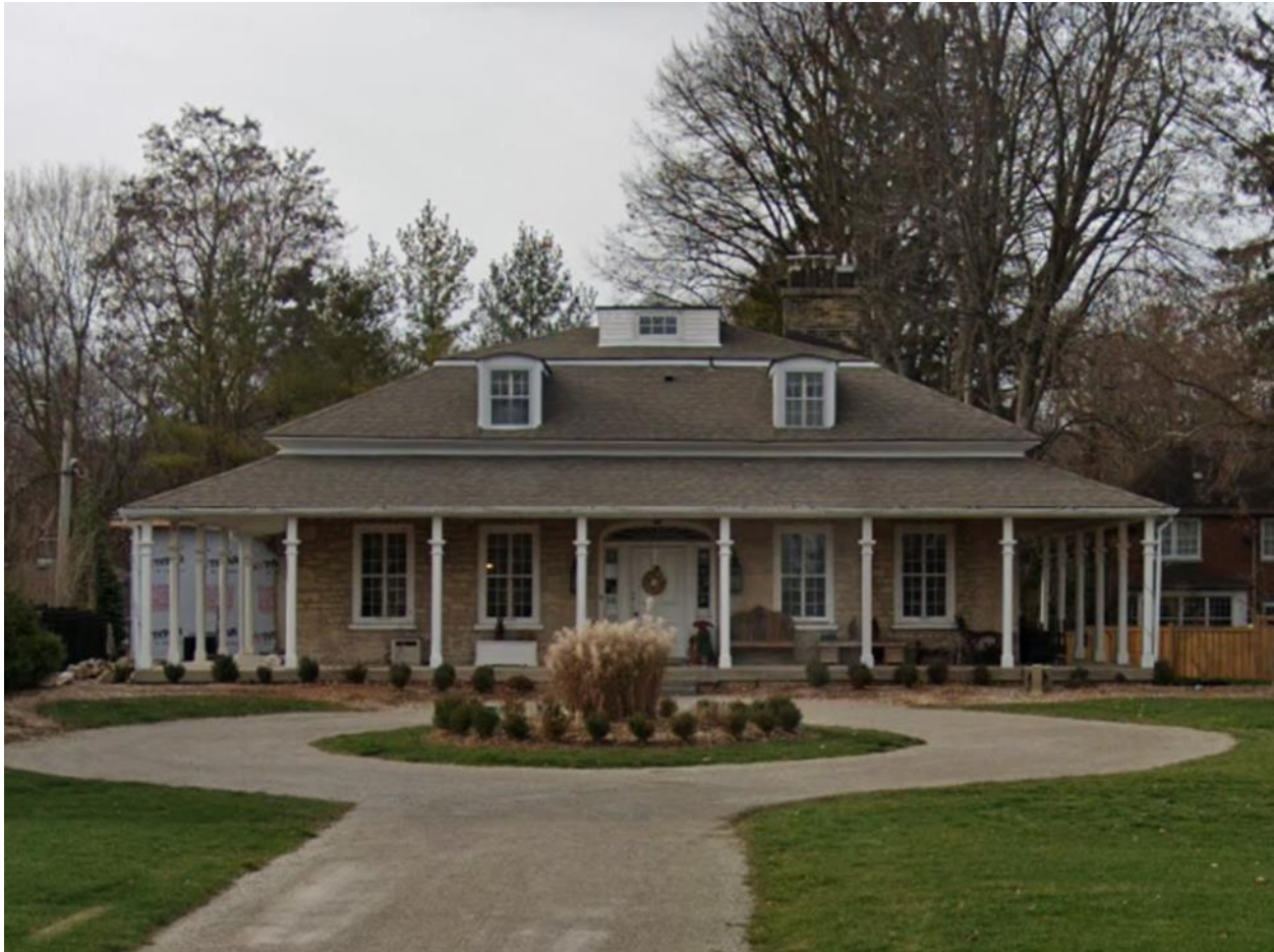
Figure 1: Front elevation of 16 Byng Avenue (Google Maps, December 2022).
