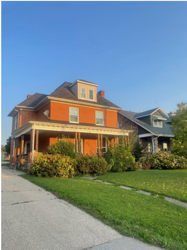
Figure 12: Front façade of 154 Beverly Street
