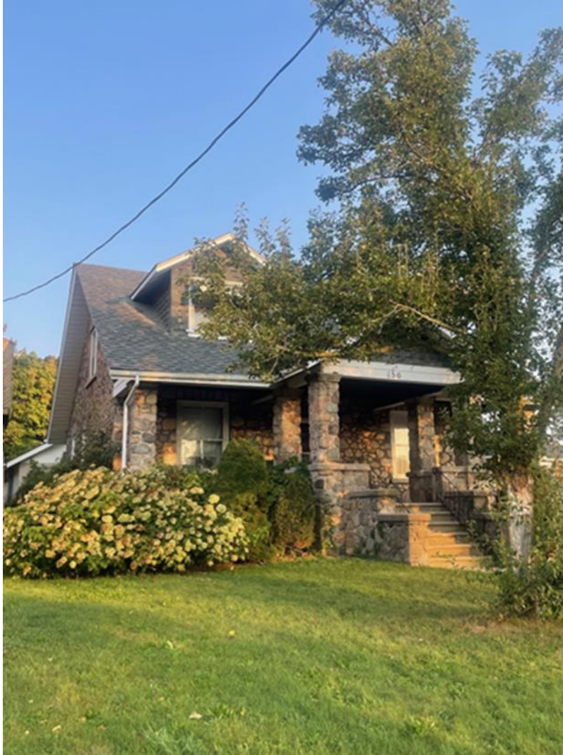
Figure 1: Front elevation of 156 Beverly Street (Scott Abbott, City of Cambridge)
