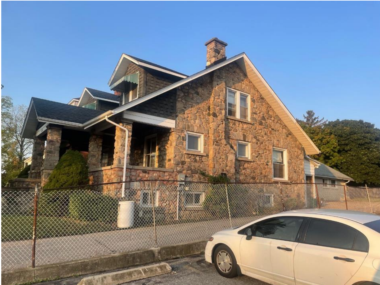
Figure 7: North Façade of 154 Beverly Street (Scott Abbott, City of Cambridge)
