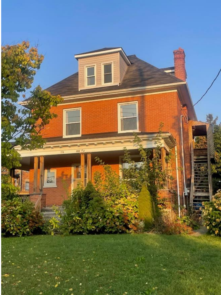
Figure 2: Front elevation of 154 Beverly Street (Scott Abbott, City of Cambridge)
