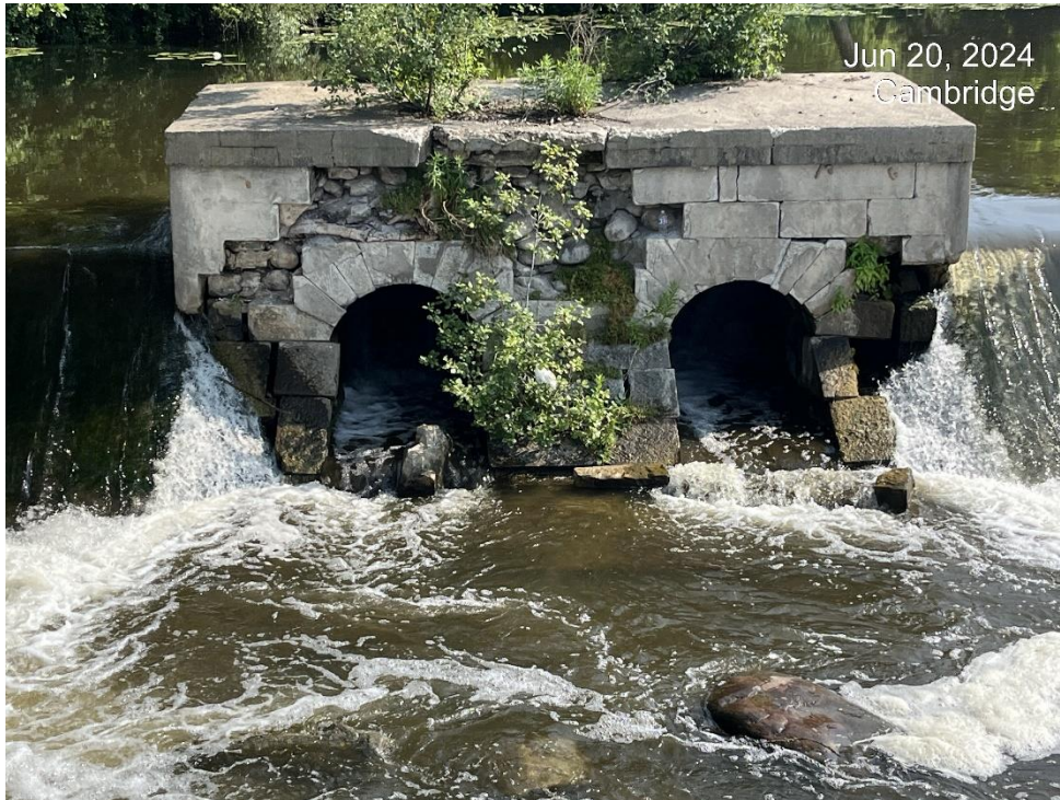
Photo 1 - Elevation View of North Stop Log Structure
