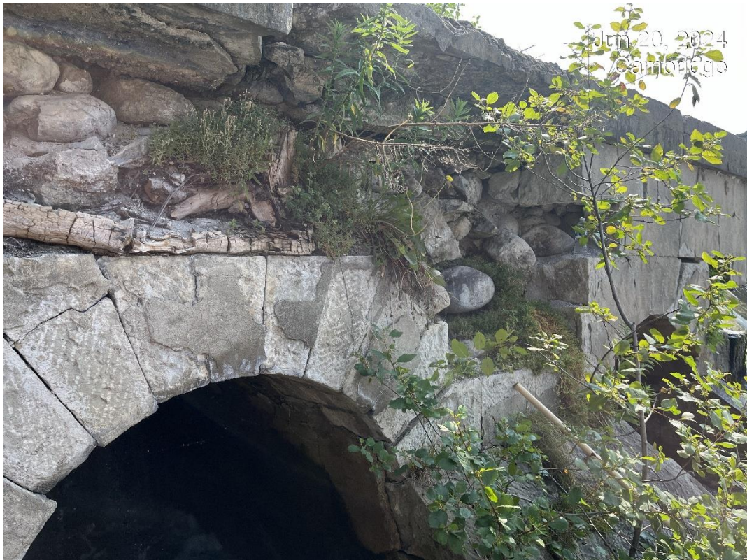
Photo 4 – Face of North Stop Log Structure
