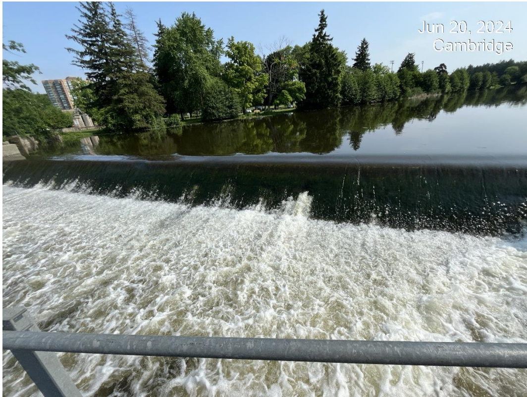
Photo 11 – Typical Condition of Spillway – Note White Water Presence due to Erosion/Spalling
