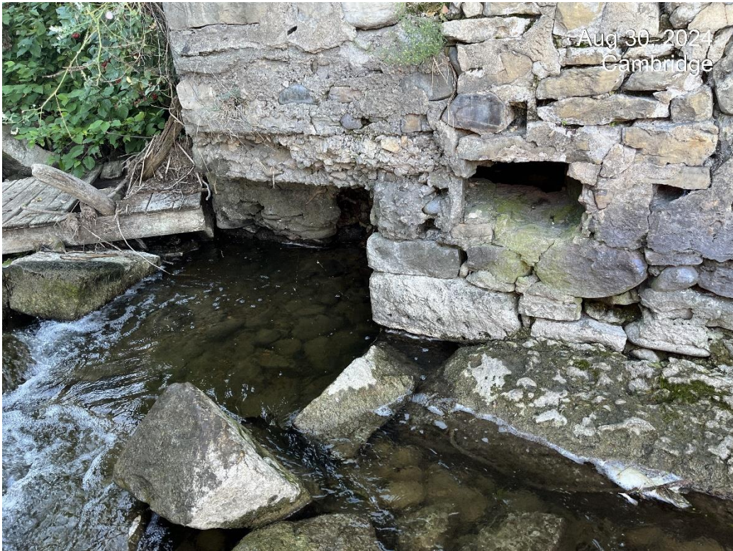
Photo 13 – South Retaining Wall – Note Cavity
