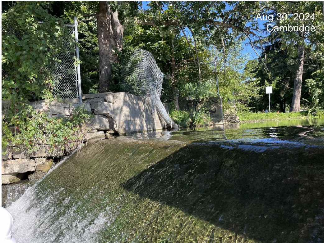
Photo 7 – North Spillway / Retaining Wall – Note Gaps in North Wall
