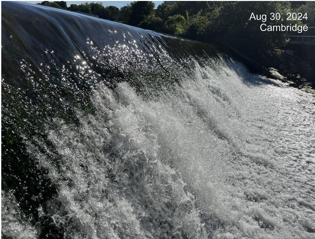
Photo 9 – Typical Condition of Spillway – Note White Water Presence due to Erosion/Spalling
