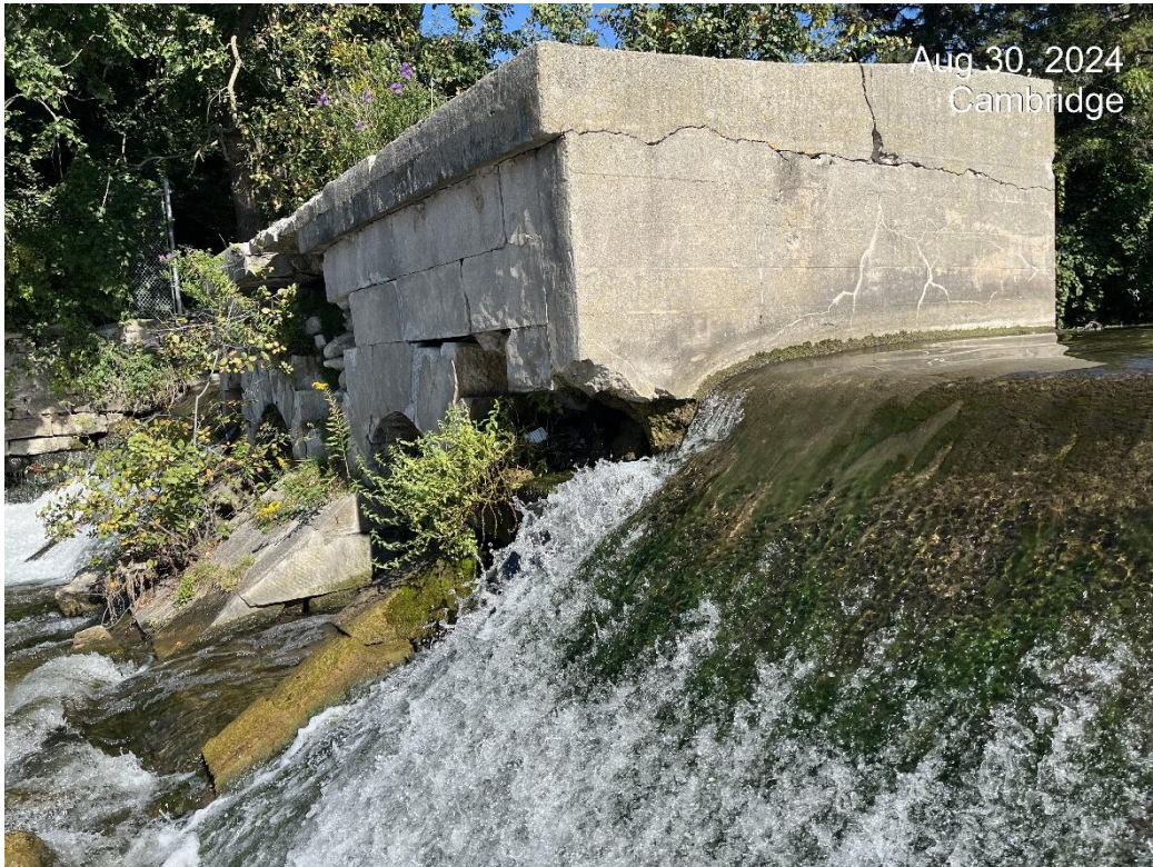
Photo 5 – Cracking along Top of North Stop Log Structure
