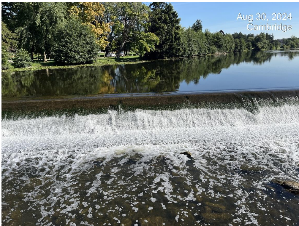
Photo 10 – Typical Condition of Spillway – Note White Water Presence due to Erosion/Spalling
