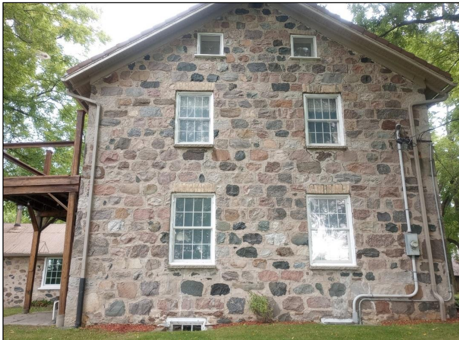
Figure 8: The east elevation (City of Cambridge).
