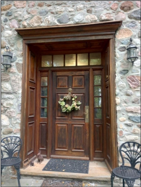
Figure 6: The recessed wooden entrance surround (City of Cambridge).
