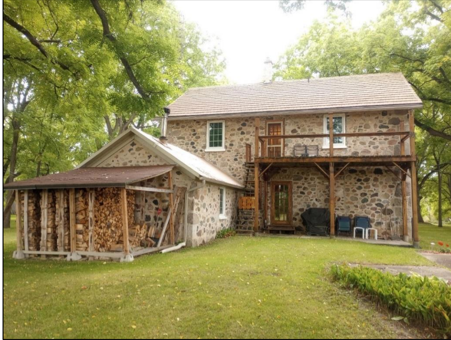
Figure 7: The rear (north) elevation showing one-storey stone kitchen tail (City of Cambridge).
