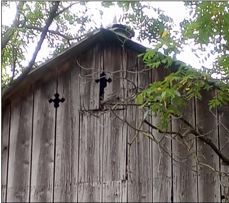
Figure 10: Cross motif cutouts visible along barn rooflines (City of Cambridge).
