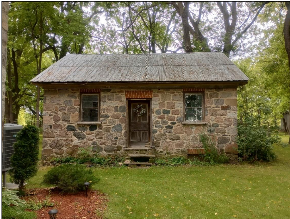
Figure 4: Facing east, view of the façade of the cook house (City of Cambridge).
