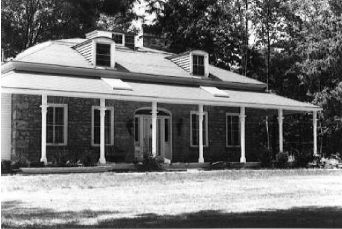
Photo 3: Front Elevation 1982 (City of Cambridge Archives).
