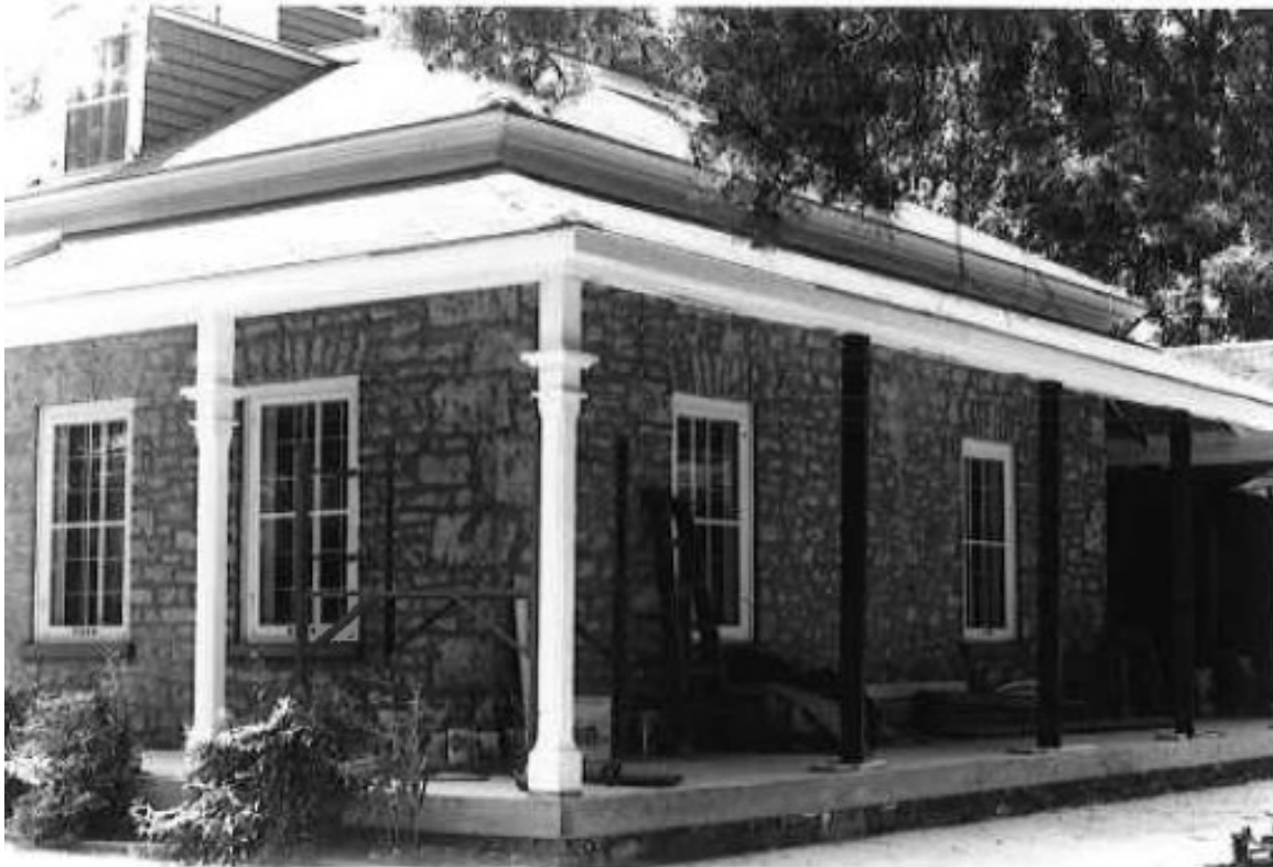
Photo 4: Side Elevation 1982 (City of Cambridge Archives).
