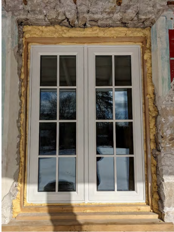
Figure 17: View north of new vinyl window, located on south elevation
