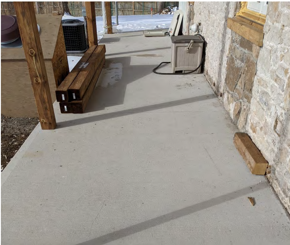
Figure 16: View west of south elevation, new cement porch
