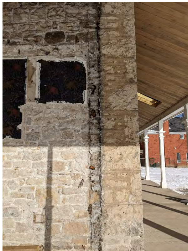
Figure 14: View north of South elevation, evidence of former kitchen and bathroom walls
