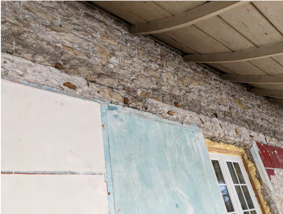
Figure 15: View north of south elevation, former kitchen and bathroom walls
