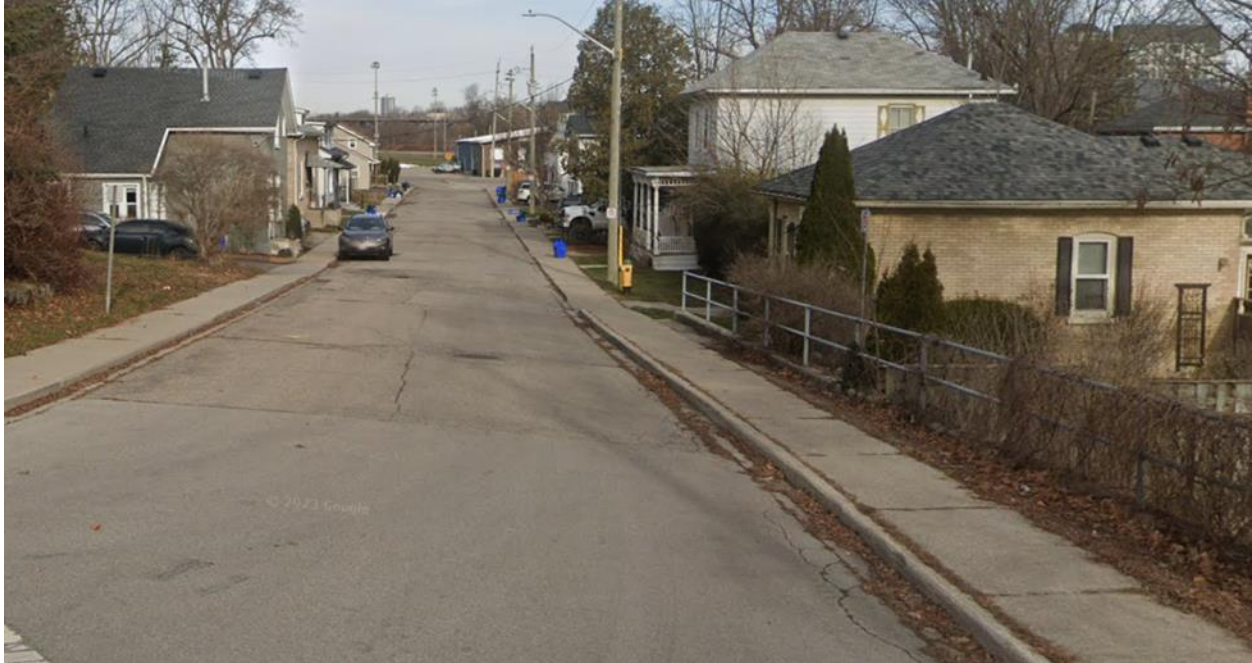
Figure 2: View of Metcalfe Street from Blair Road in the Dickson Hill HCD
