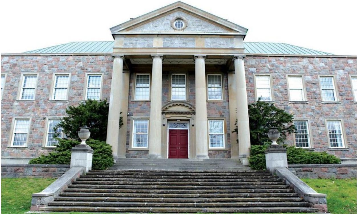
Figure 1: Front elevation of 252 Dundas Street North (Cambridge Times).
