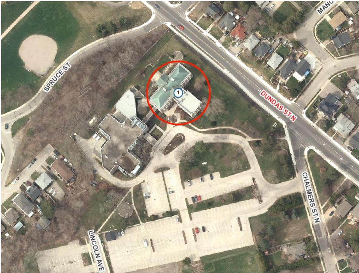
Figure 4: The Gore Mutual building outlined in red on aerial image (City of Cambridge).
