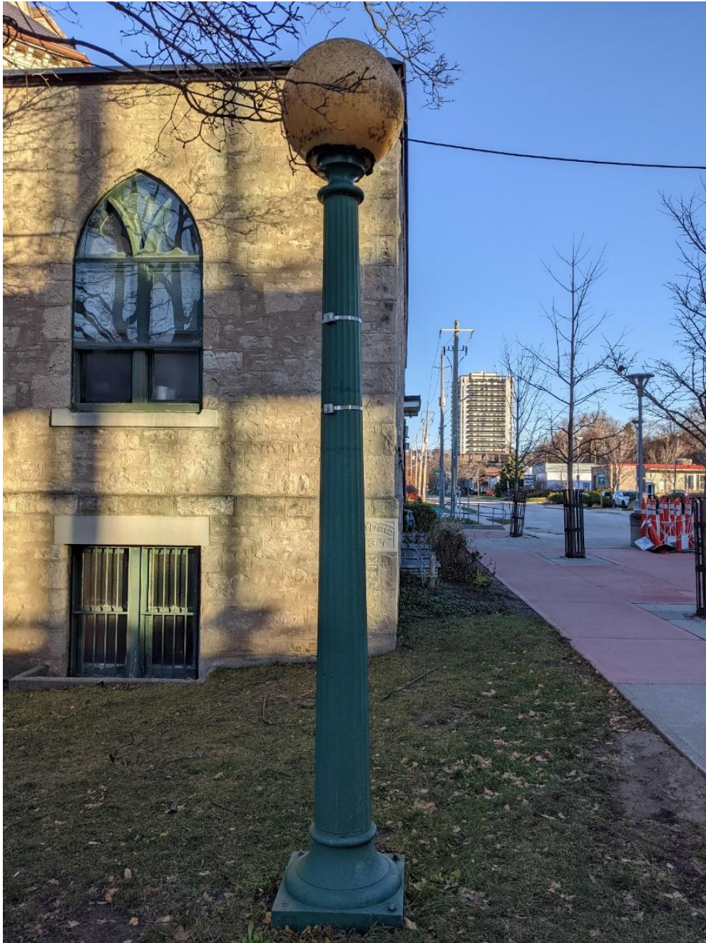
Figure 1: Existing Decorative Globe Light Pole, December 13, 2021.
