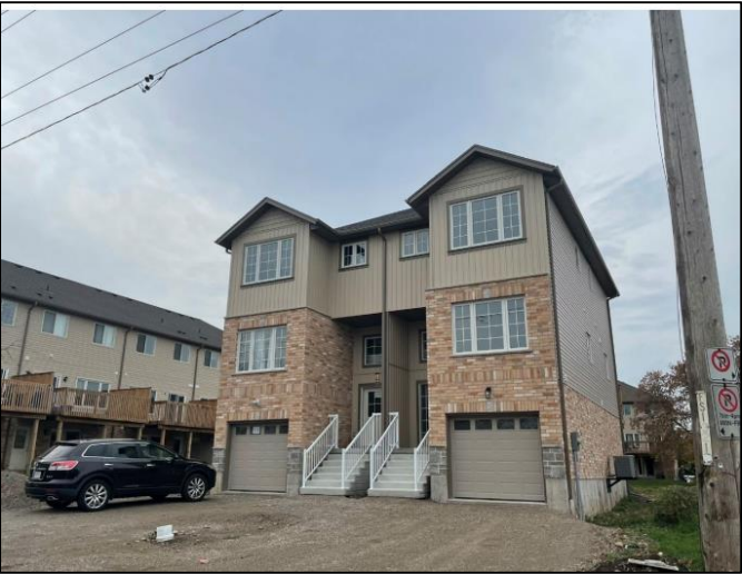
Figure 3 – Existing semi-detached at 214 and 216 Union Street North
